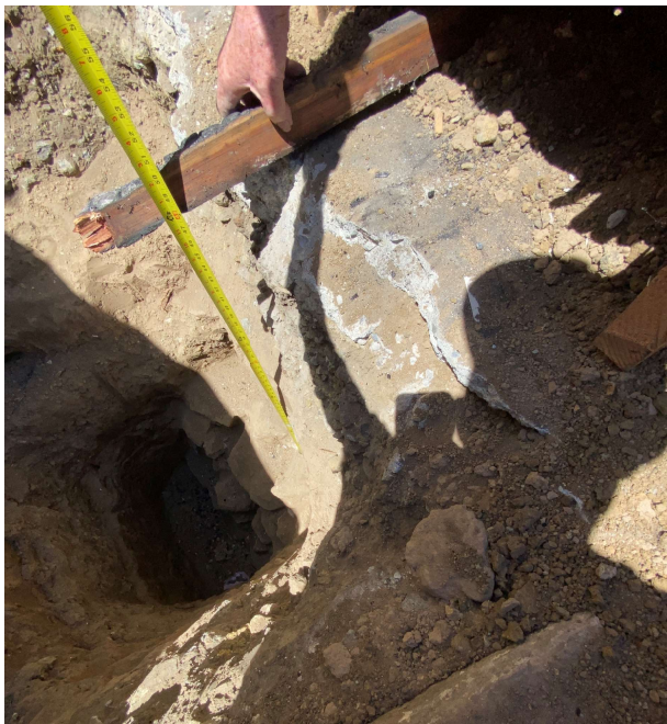
Top of Grade to Top of Culvert - 48"
