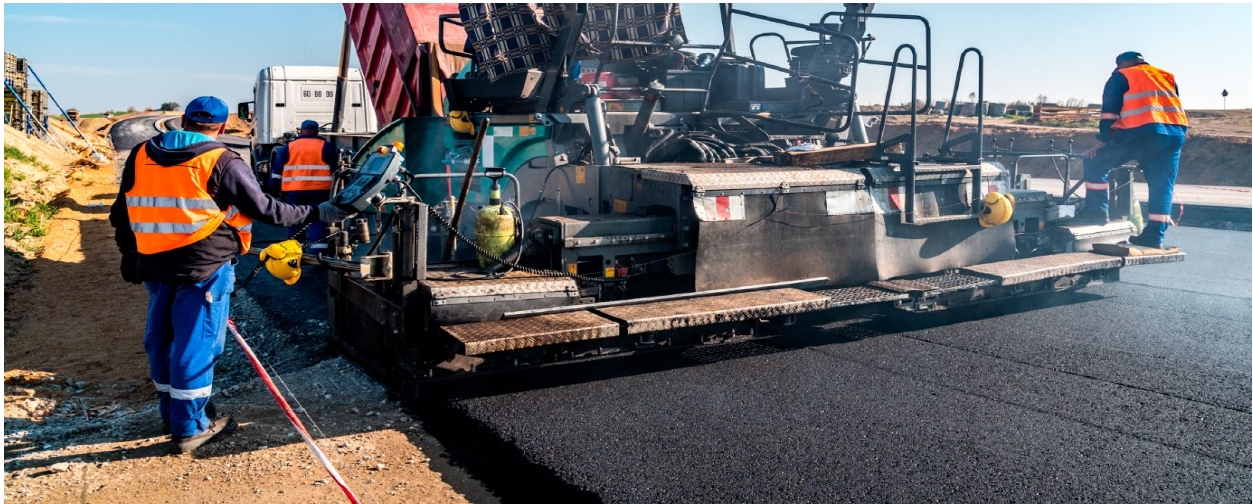
Pavement Upgrades, Byron Highway
