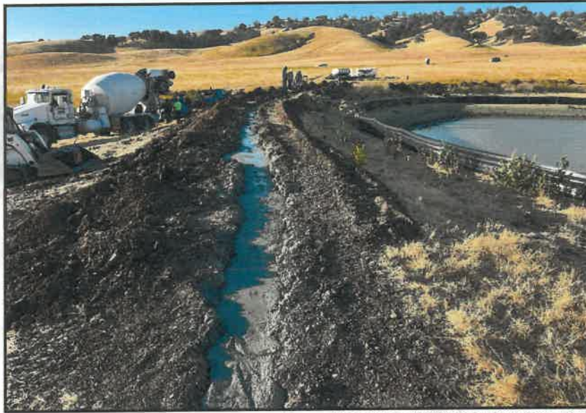
Concrete slurry trench
