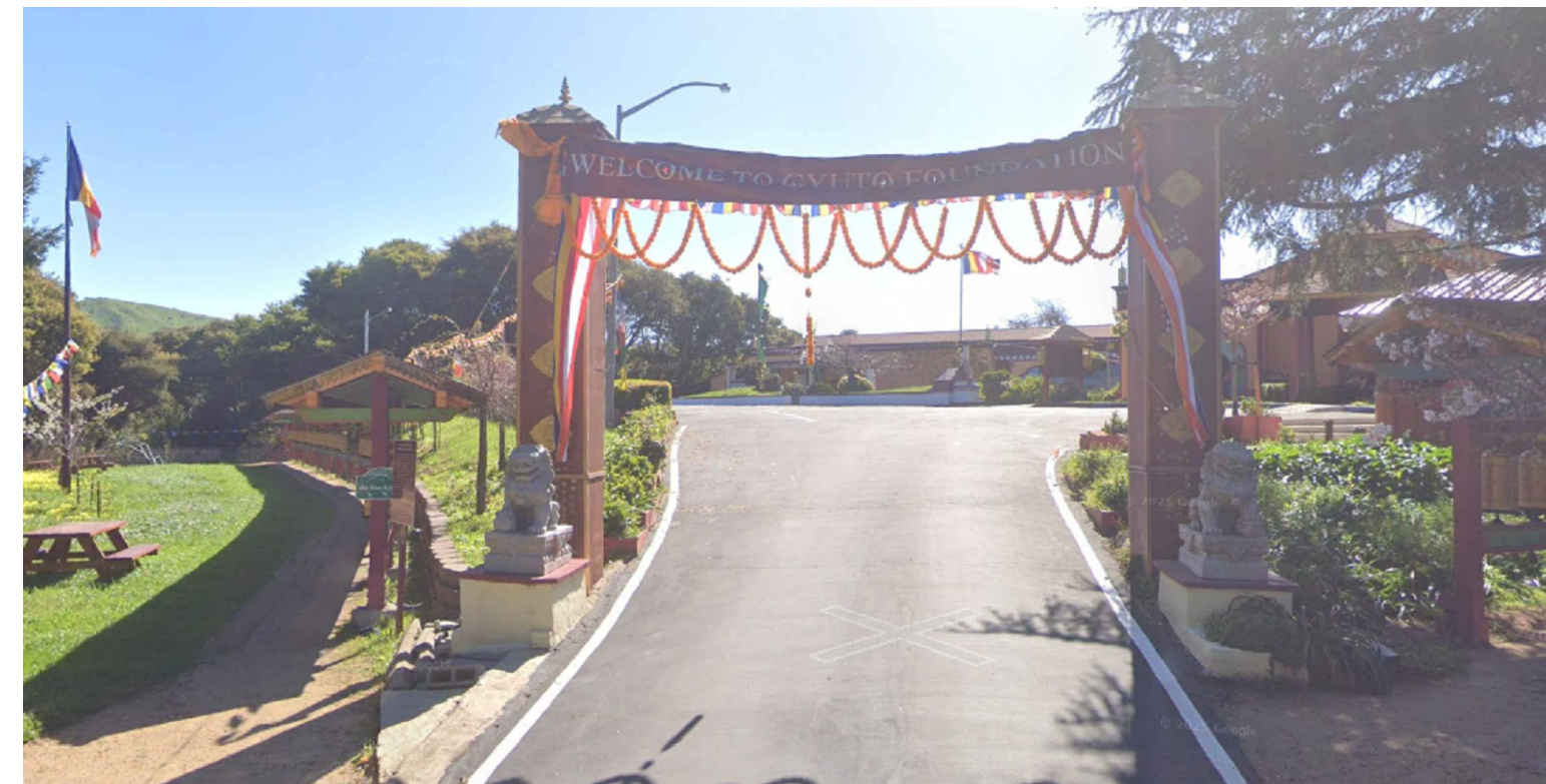
EXTERIOR OF SECONDARY GATE TO REMAIN AS IS. IT IS RENOVATED BY WOODEN POST WITH PLASTER FINISH.
