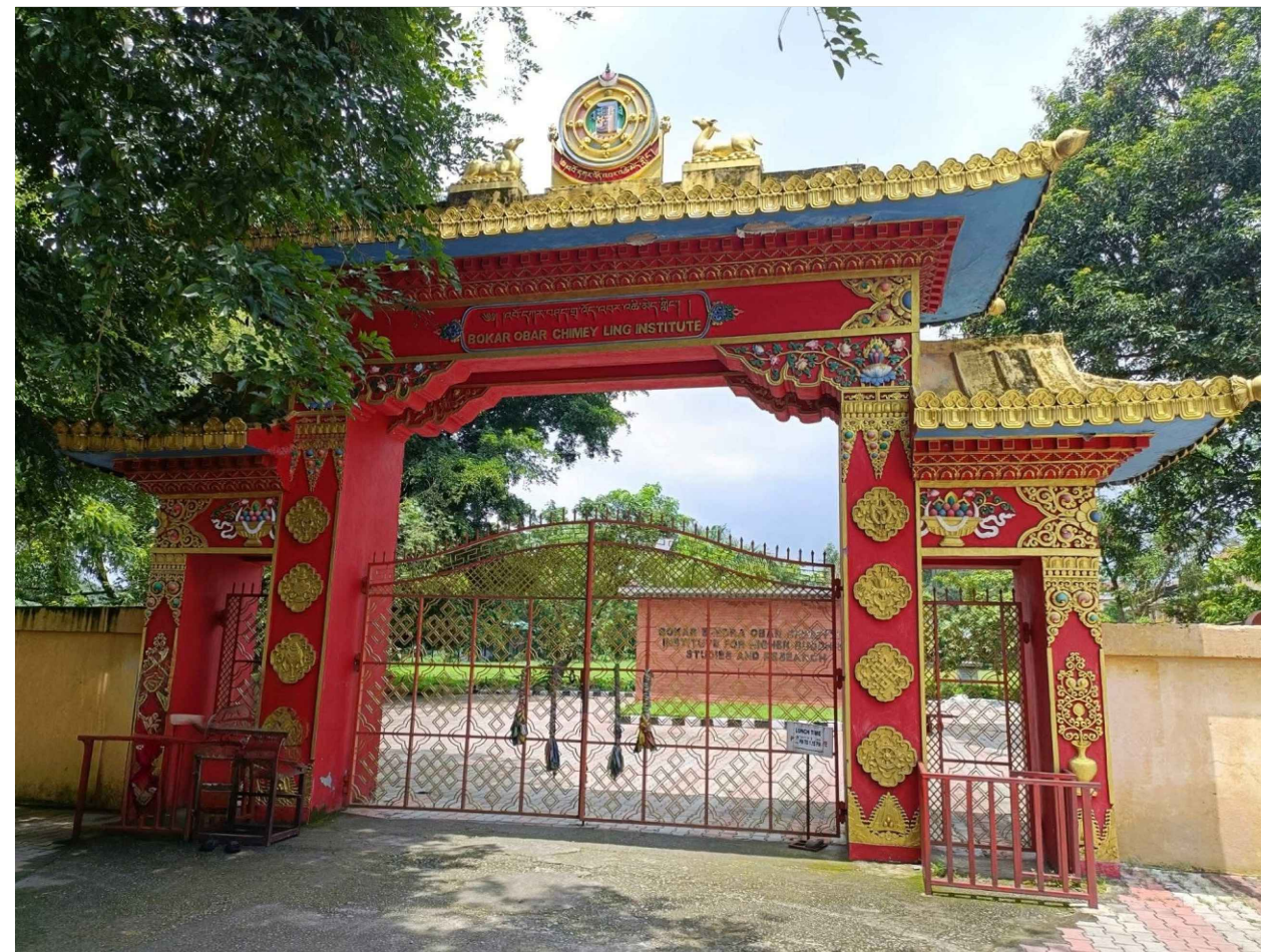
REFERENCE PHOTO FOR MAIN GATE
