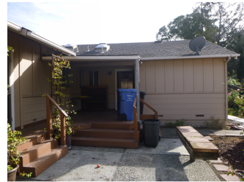
REAR DETAIL - PORCH
