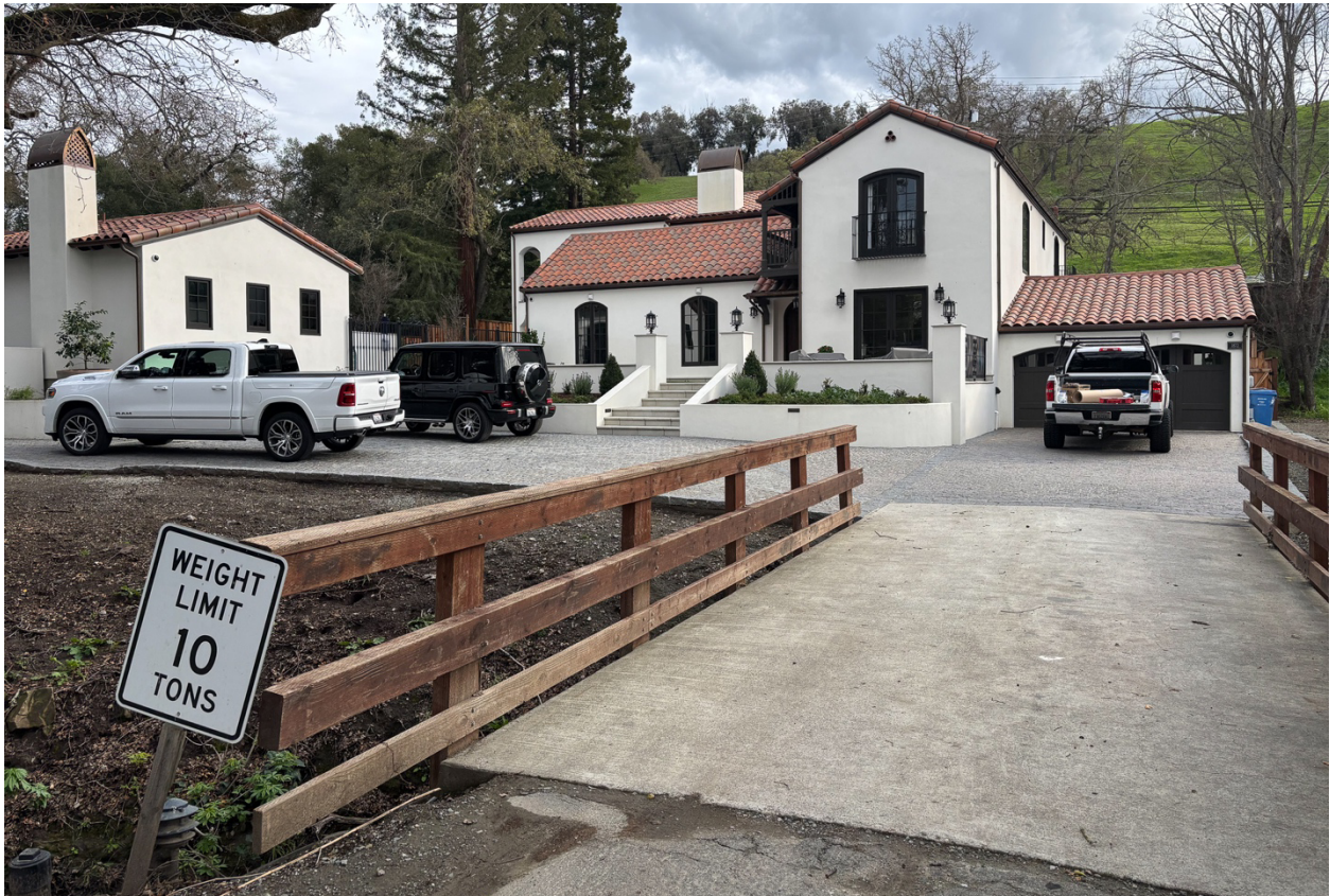
Fig.7 – 1872 Alameda Diablo – Front from driveway & bridge
