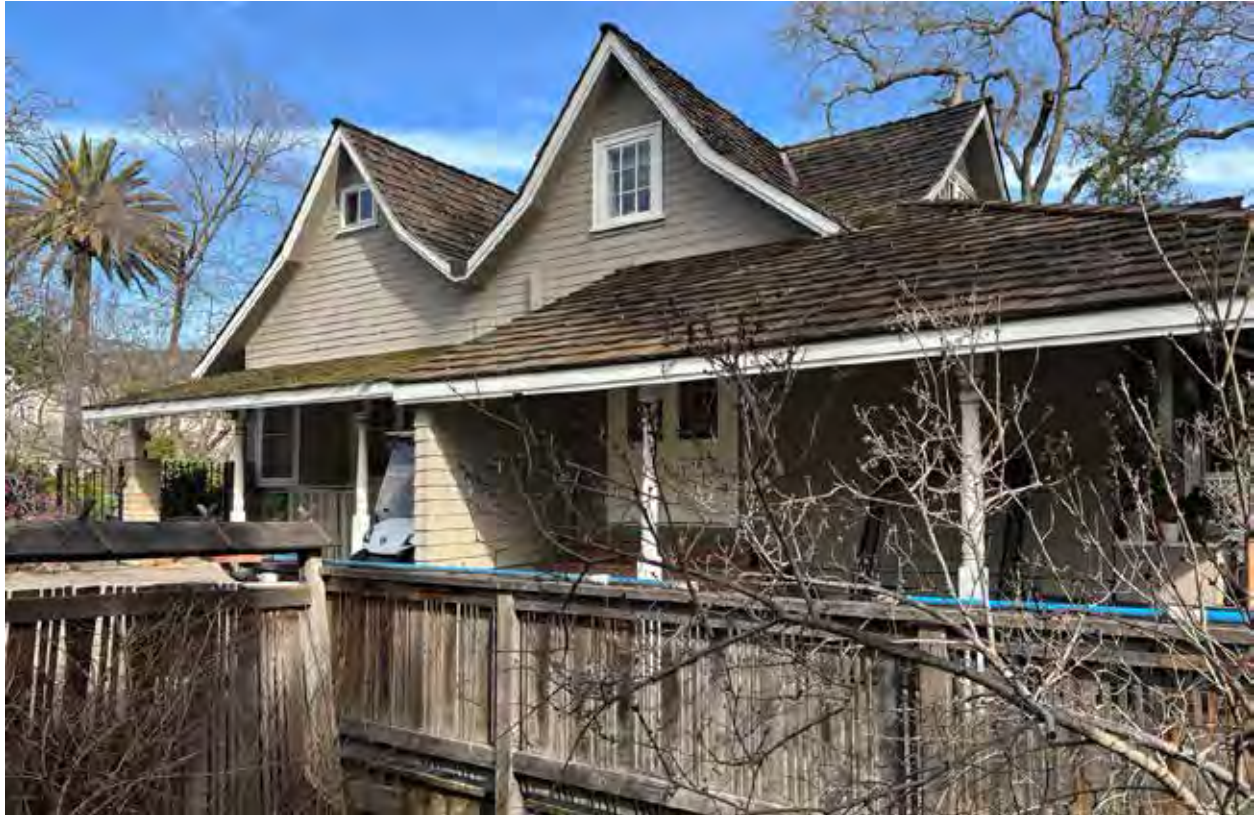
Fig.13 – 1850 Alameda Diablo – West side from creek bridge
