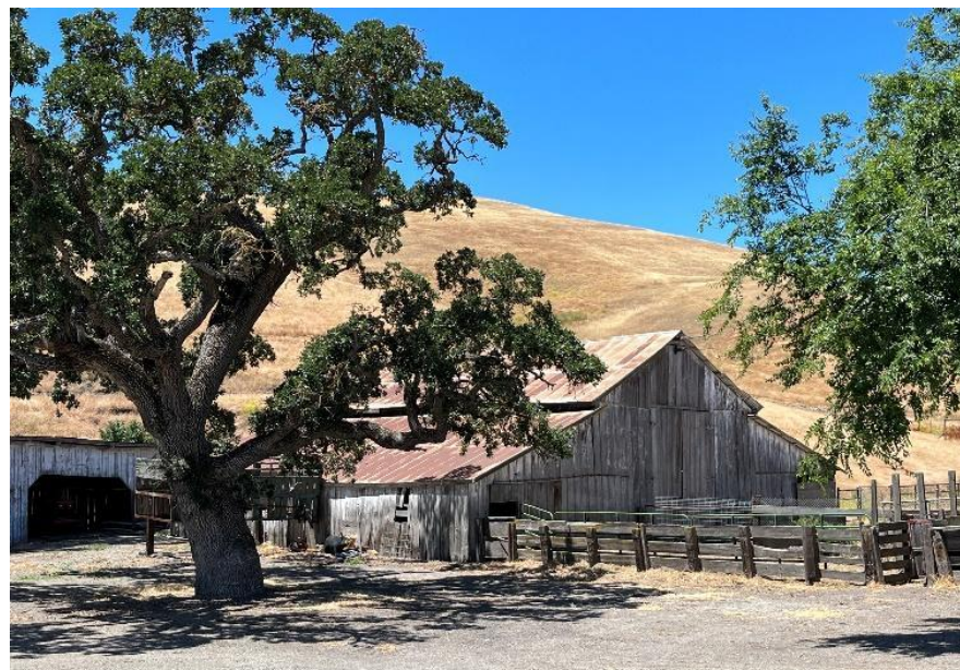
Agricultural buildings, like this barn in Tassajara Valley, enhance the character of rural areas.
