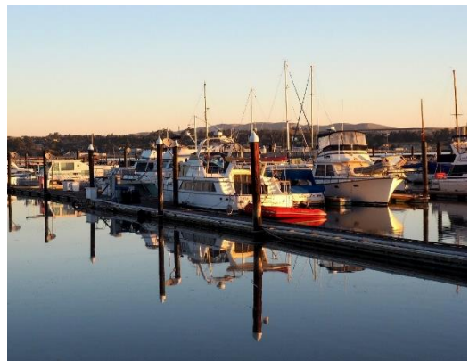
Shoreline facilities, such as this marina, are at particular risk from shoreline flooding. Photo credit: Lisa Gorrell.
