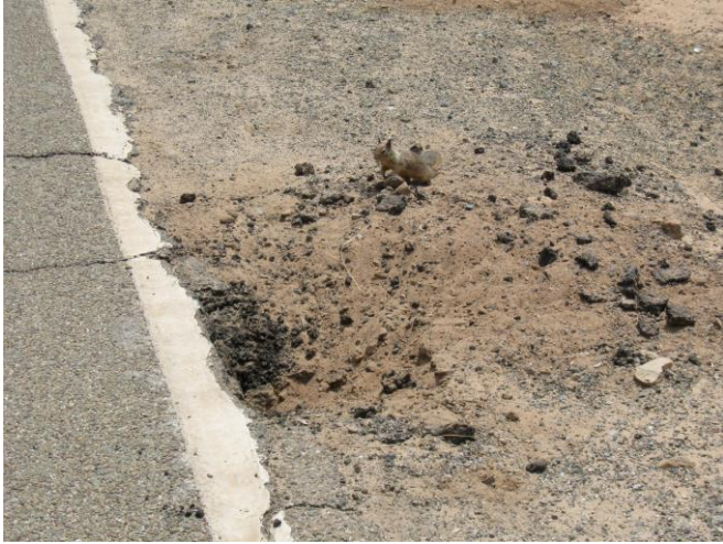
Ground squirrel and burrow under Empire Mine Road near Antioch in eastern Contra Costa County
