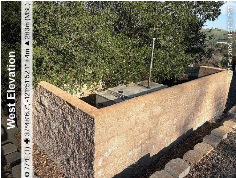
COA 19 Generator enclosure CMU wall in lieu of wood fence for durability
