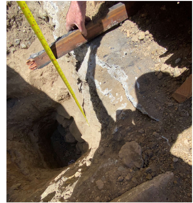
Top of Grade to Top of Culvert - 48"
