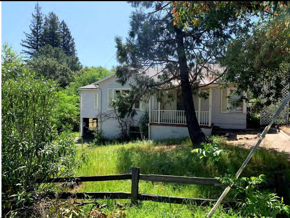
1. Photo taken facing south showing the two-story residential home and surrounding woodland habitat at northwestern boundary of Property. Photo taken April 6, 2021.
