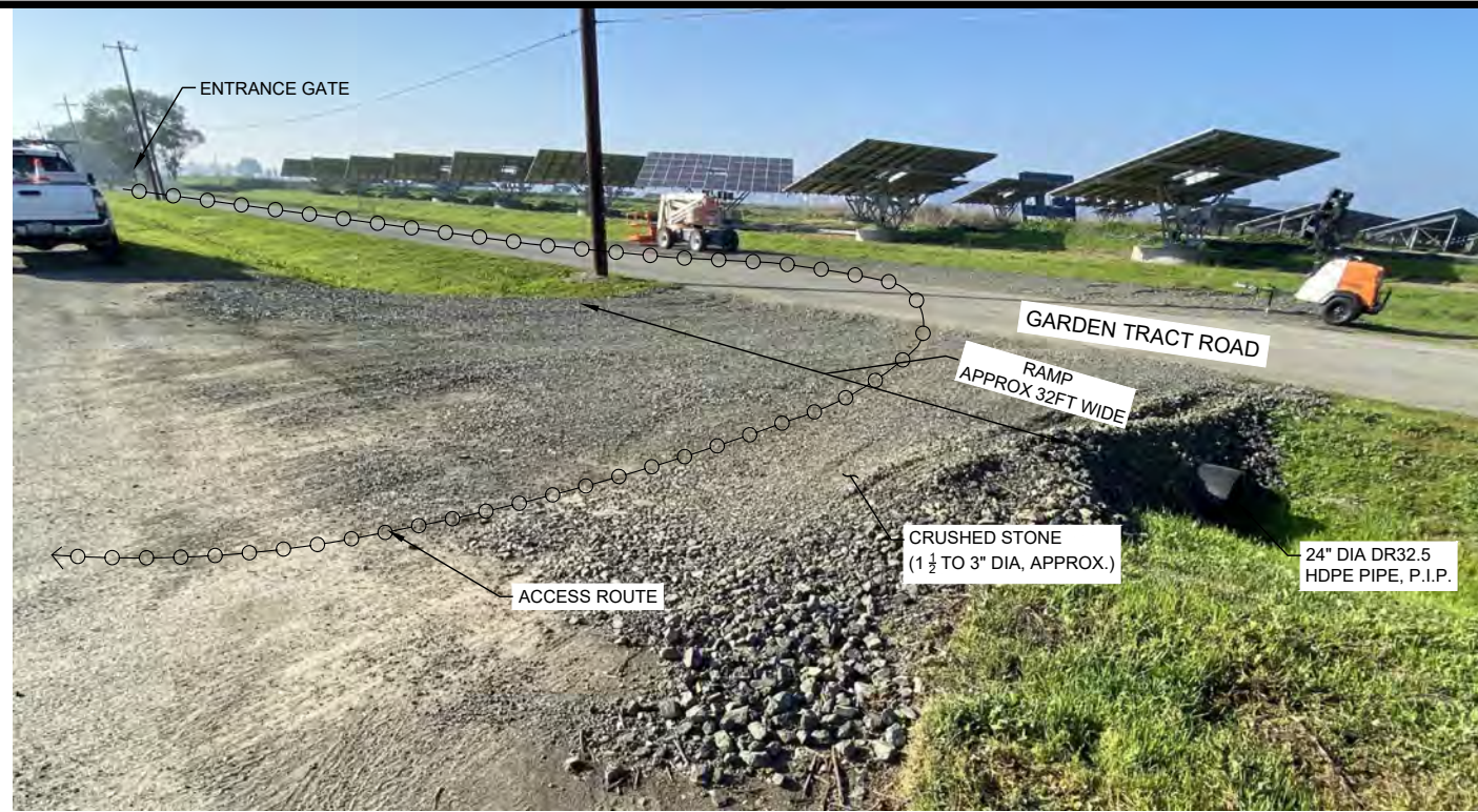
PHOTO 2 ACCESS RAMP G-1 PHOTO N.T.S.
