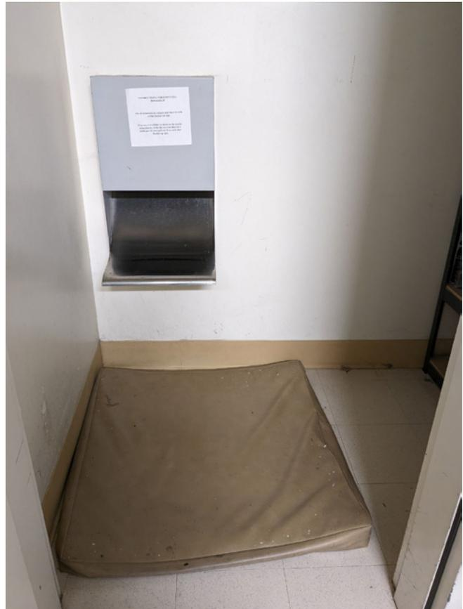
An example of adequate clearance not being provided for a bin below the book drop. A cushion was placed on the floor to receive the dropped books, which must be collected up by staff (an ergonomic issue).
