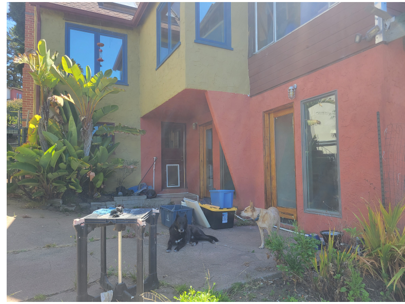
4. AREA IN FRONT OF (E) LOWER LEVEL DOORS SHOWING OLD (E) DRIVEWAY
