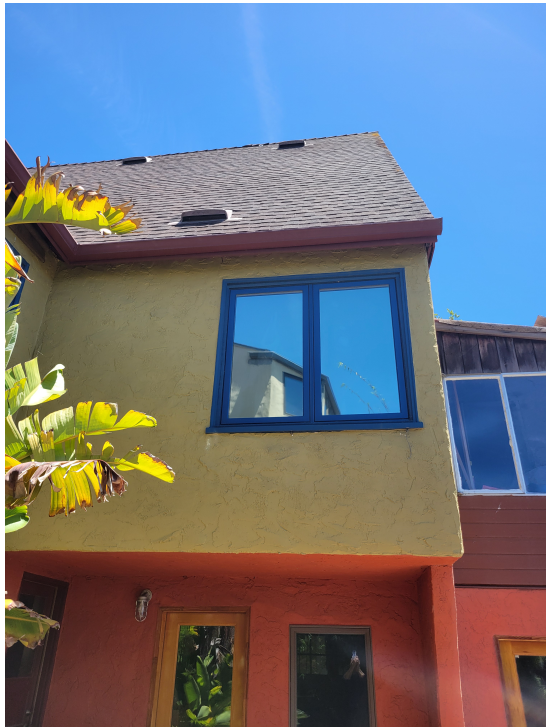
3. ROOF WHERE BEDROOM DORMER WILL GO.
