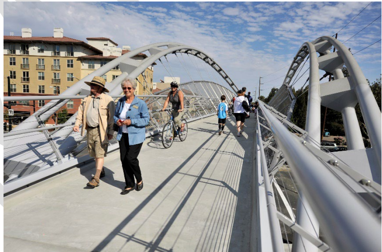
Contra Costa Centre Overcrossing
