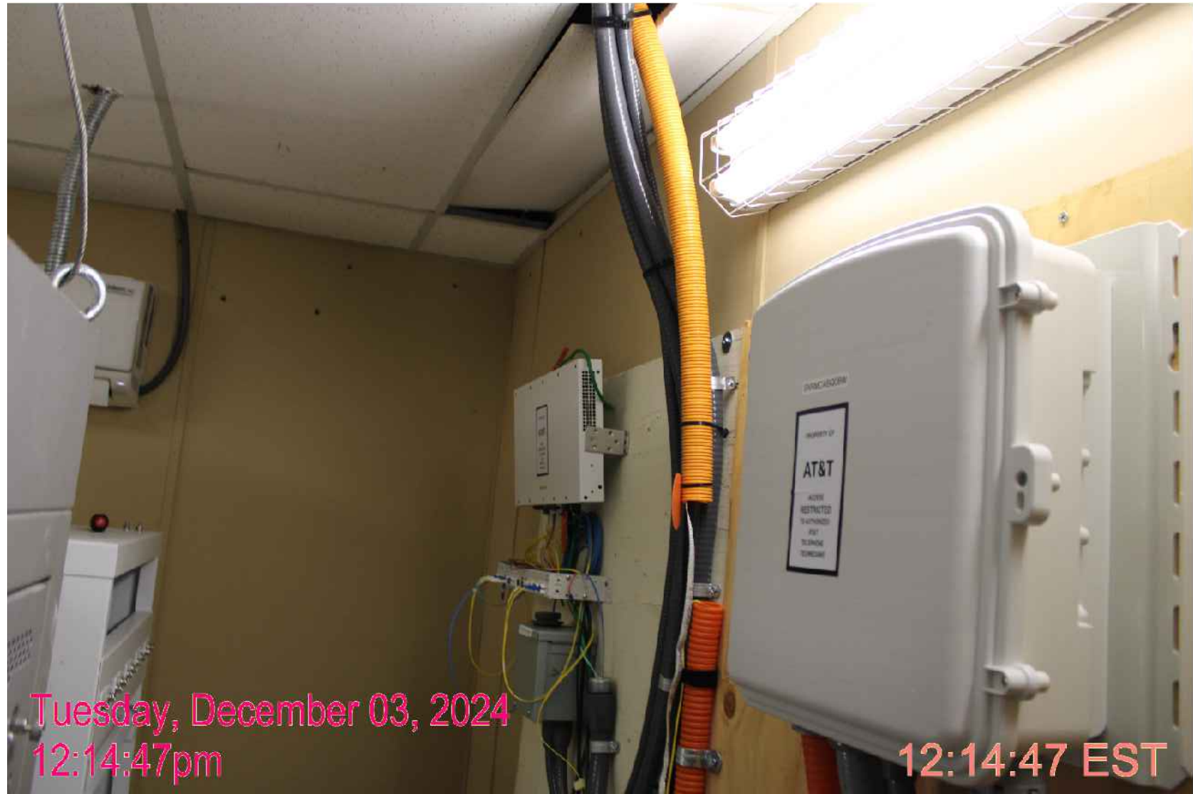
FIBER CEINA BOX AND AAV BACKBOARD
