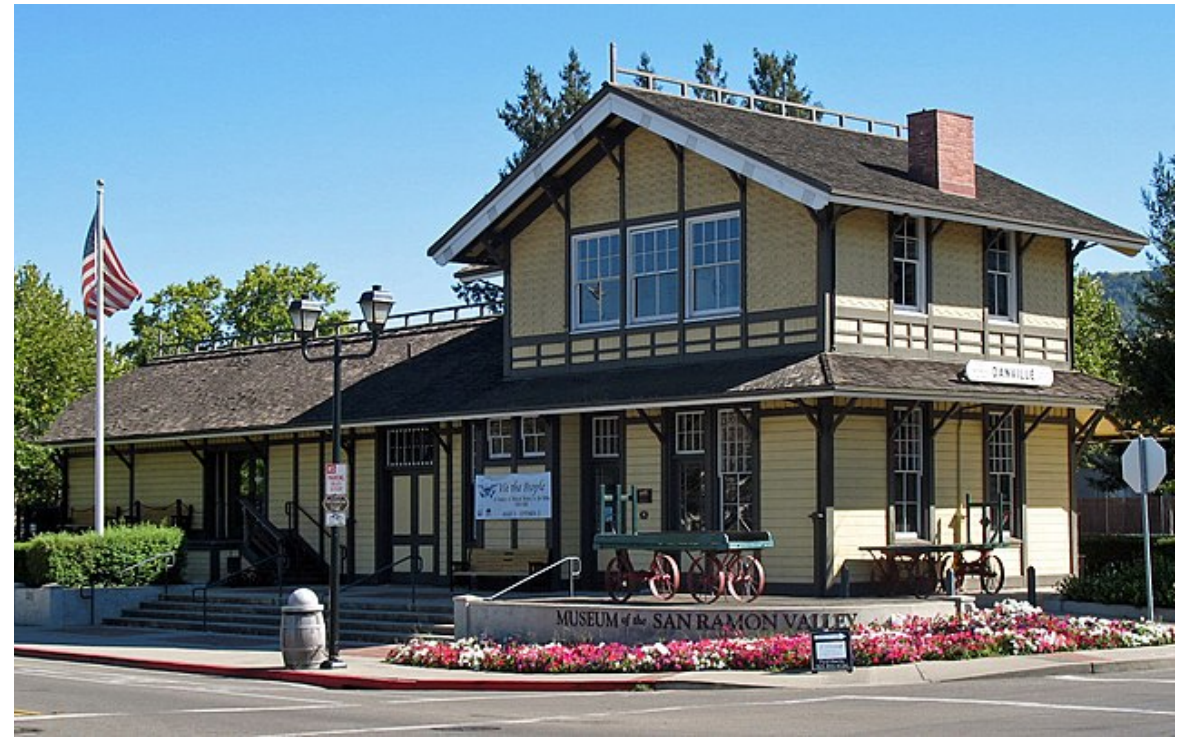
Danville Railroad Depot (1891), Danville
