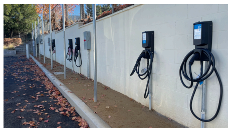
County departments are investing in electrifying their fleets; for example, these Flo Level 2 electric vehicle (EV) chargers
