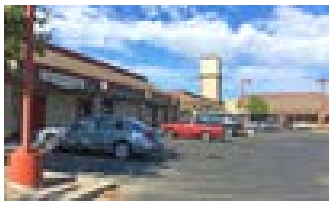
Existing shopping center in Bayview.
