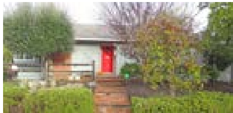
Existing single-family home in El Sobrante.
