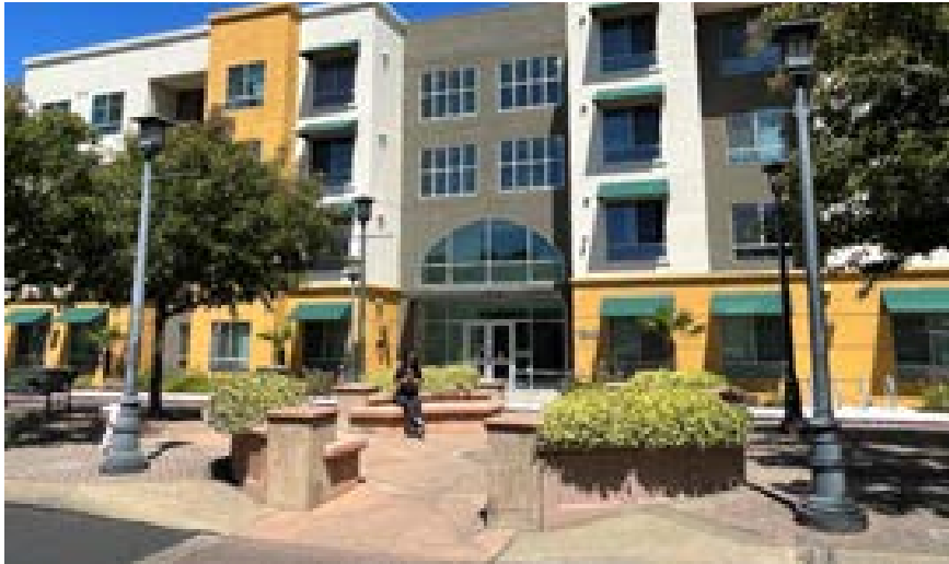
Streetscape improvements like this project along Fred Jackson Way in North Richmond are provided by the County's Public Works Department.
