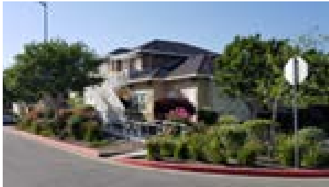
Multi-family housing in Bay Point.
