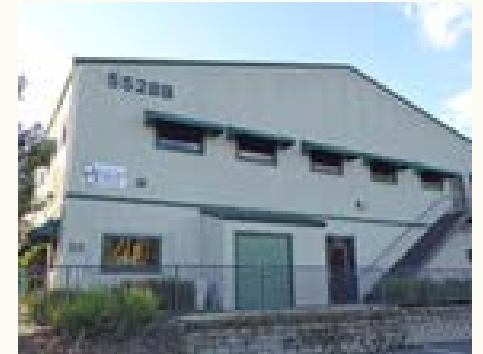
Existing office uses in Pacheco.
