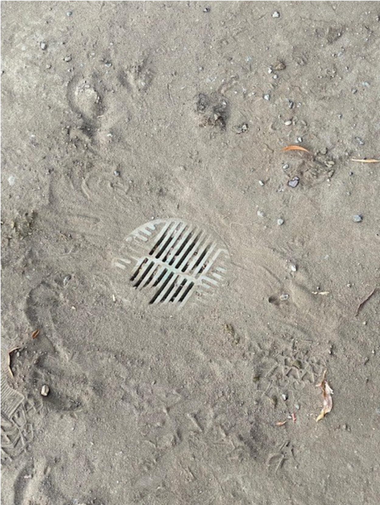
Drain pipe flush out
