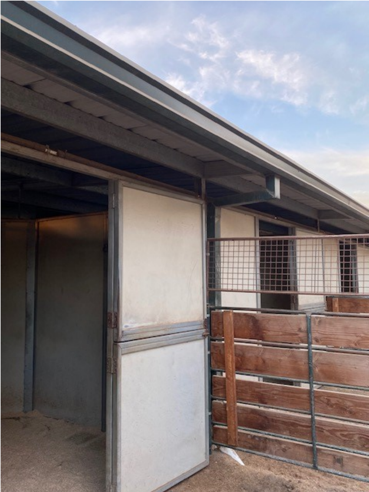
Gutters and Downspouts above paddocks
