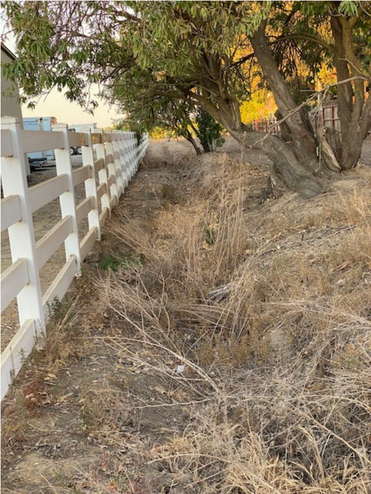
Drainage to Irrigation/Ag District runoff system
