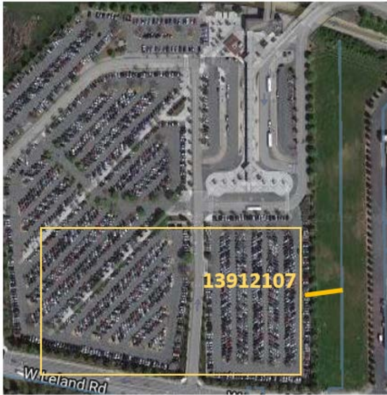
Figure 33. Pittsburg/Bay Point BART
