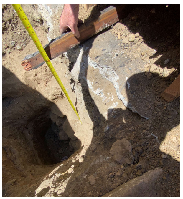
Top of Grade to Top of Culvert - 48"
