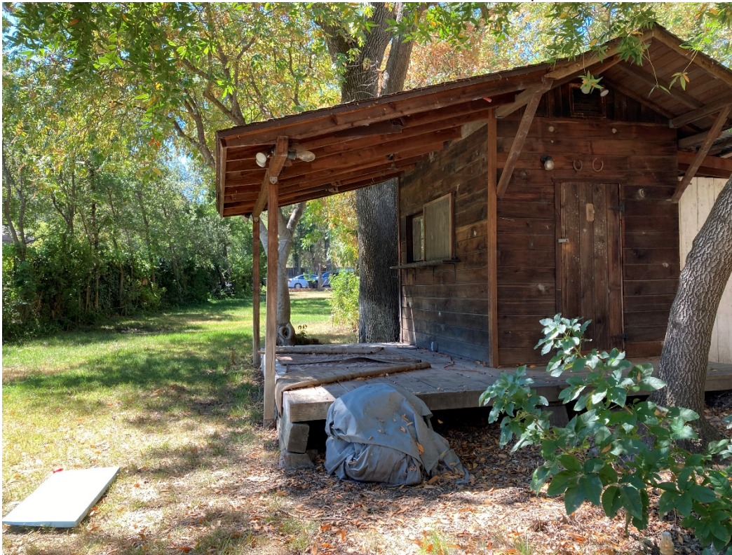
Existing shed proposed for demolition
