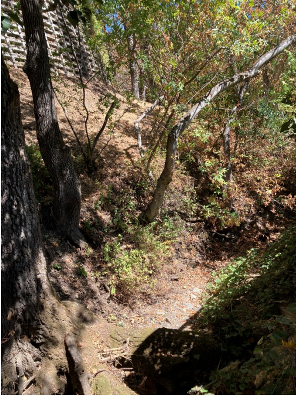
Open/daylit area of Creek
