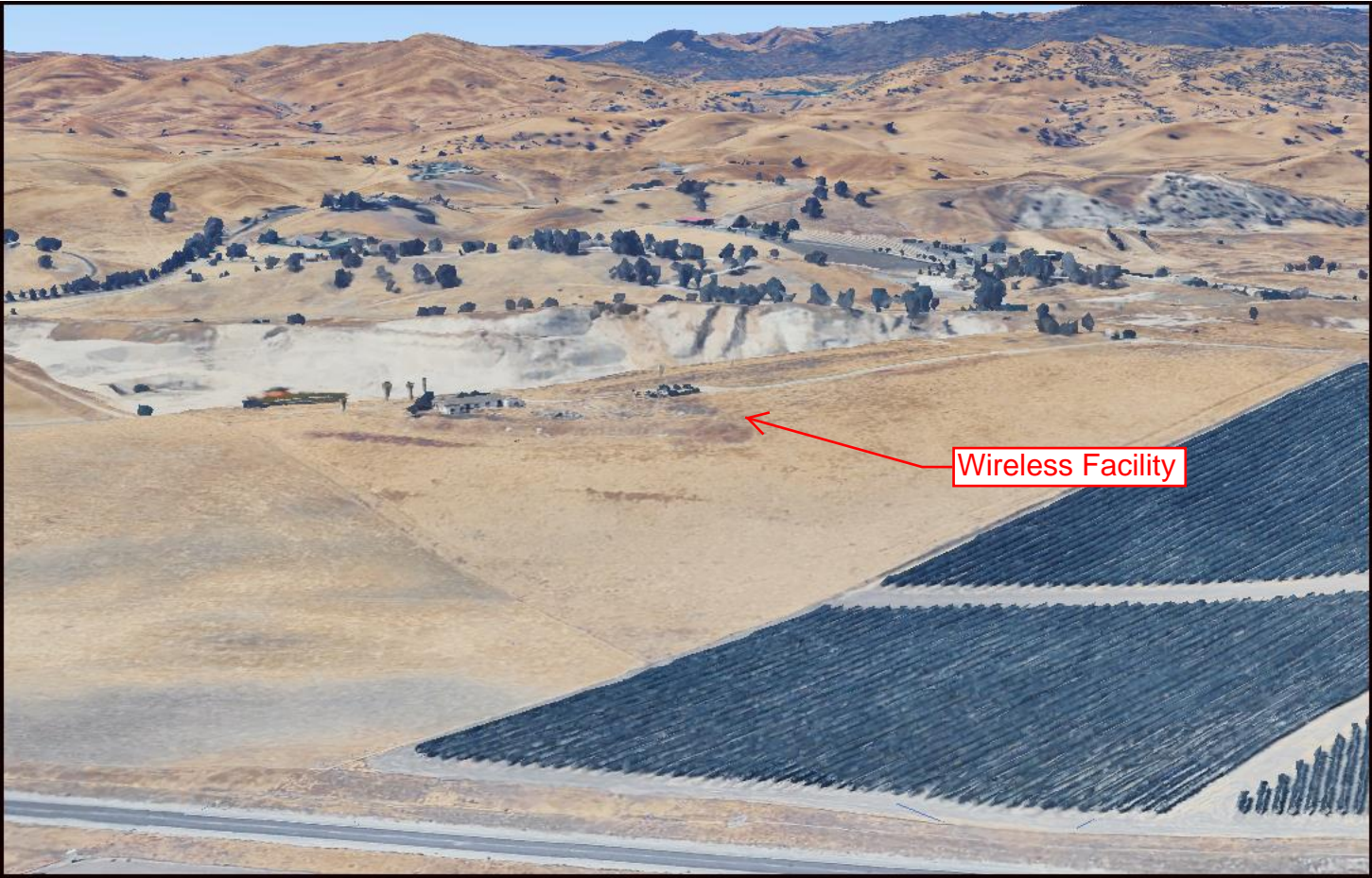
View southwest of wireless facility; Vasco Road in foreground
