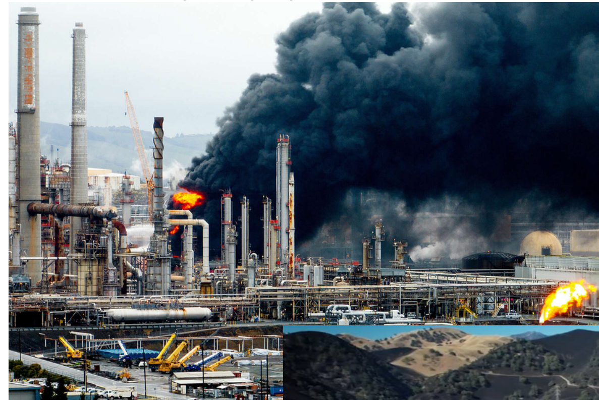
Martinez Refinery Company Fire 2/1/2025
