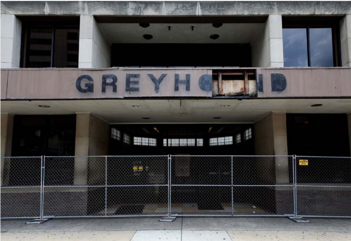
An abandoned Greyhound bus facility in Birmingham, Alabama. Photographer: Raymond Boyd/Michael Ochs Archives via Getty Images
