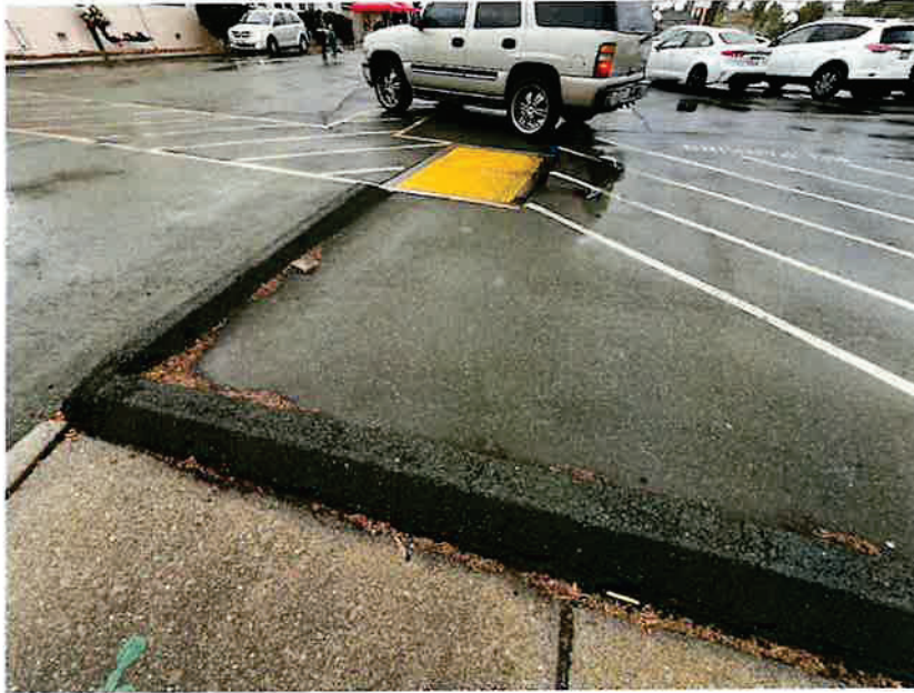
Photo 1. Southeast corner of the Oakley Elementary Parking Lot
