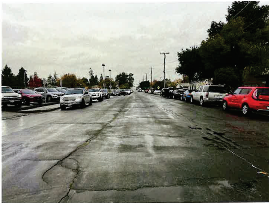
Photo 6. Norcross Lane (North Bound)
