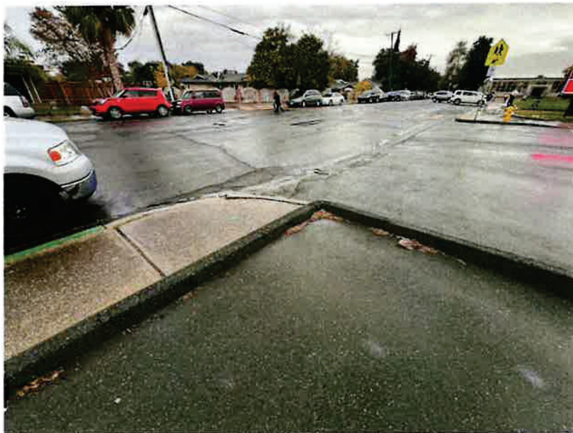
Photo 2. Southeast corner of the Oakley Elementary Parking Lot with Norcross Lane
