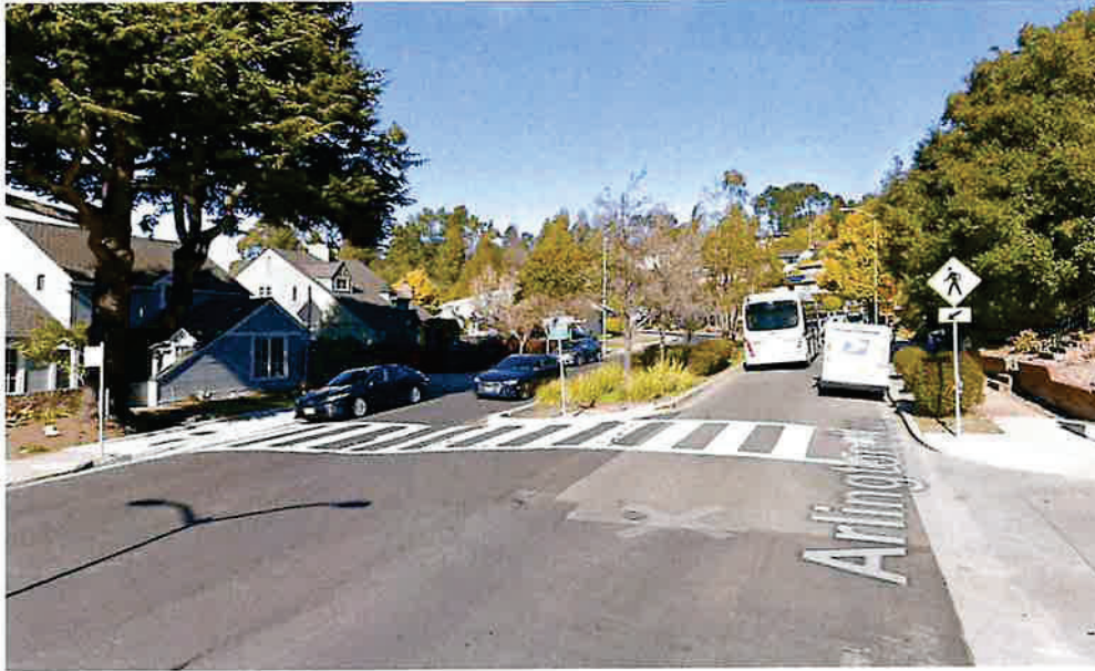
Photo 3: The crosswalk at Arlington Ave and Westminster Ave, which has a long crossing distance and visibility problems in the morning due to fog.
