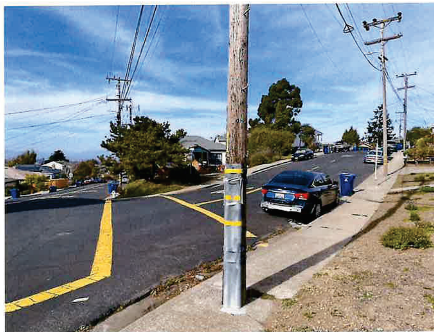
Photo 2: The crosswalk crossing Elm Ave at the intersection of Arlington Blvd and Elm Ave, with no curb ramps and a power pole in the pedestrian's path of travel.
