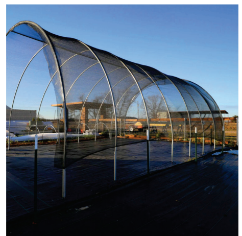
Example of a shadehouse structure. Photo courtesy of Bootstrap Farmer .
