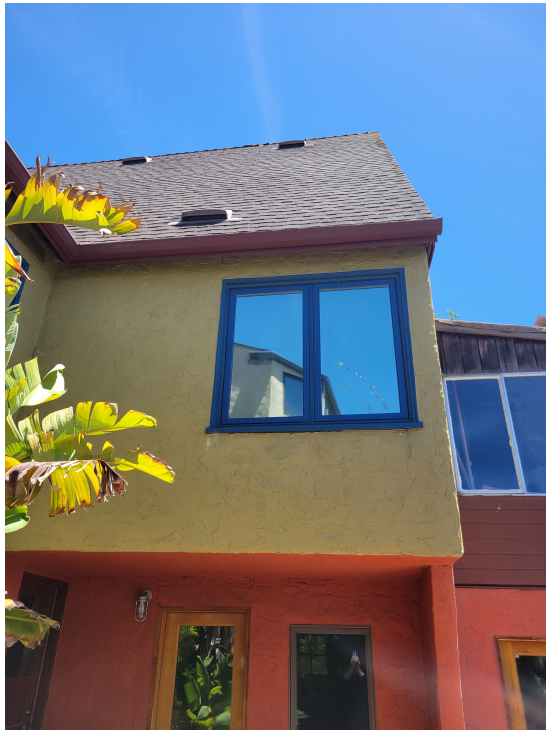
3. ROOF WHERE BEDROOM DORMER WILL GO.
