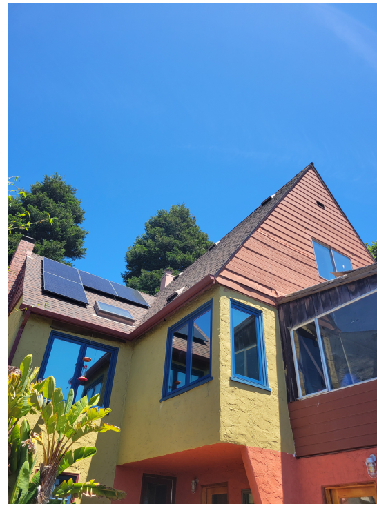
2. AREA WHERE DEN EXTENSION WILL GO
