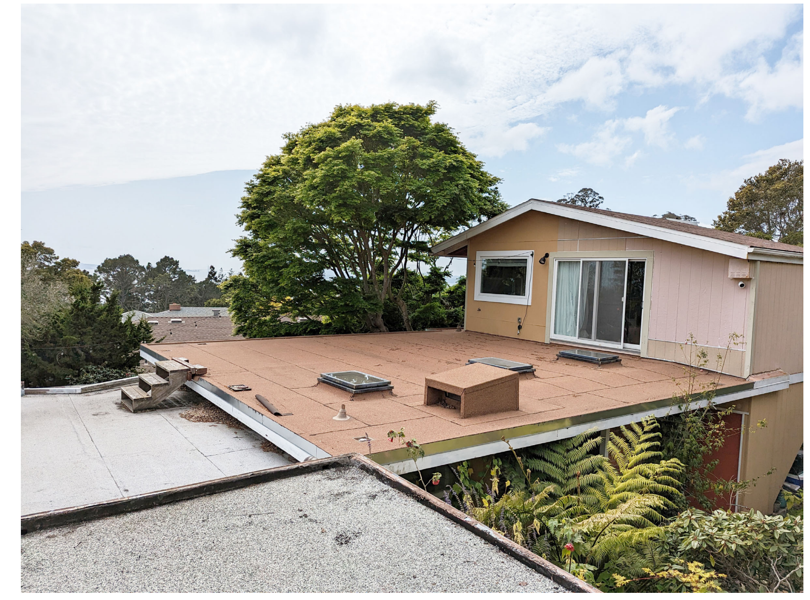
(E) ROOF @ PROPOSED MAIN DECK LOCATION
