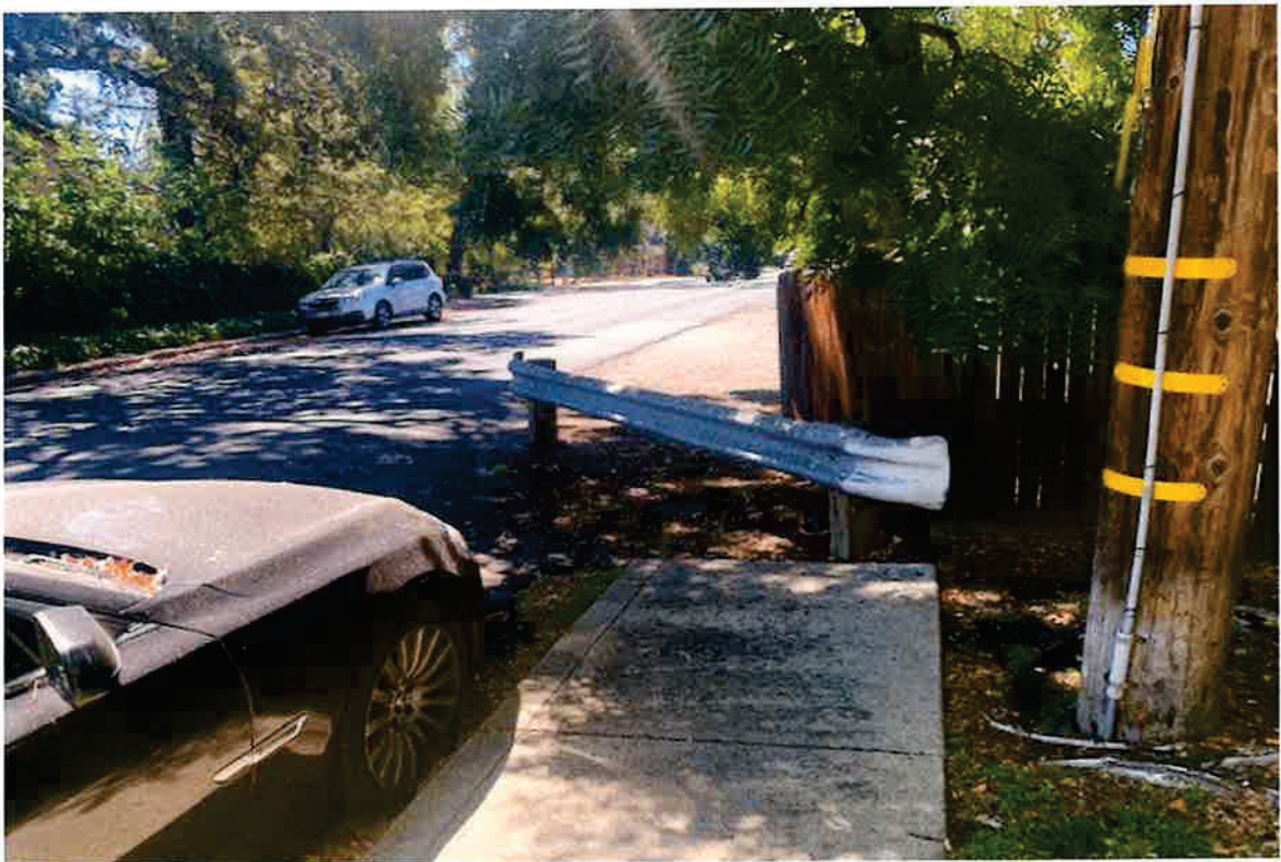
Photo 2: Mayhew Way sidewalk looking west where existing sidewalk ends
