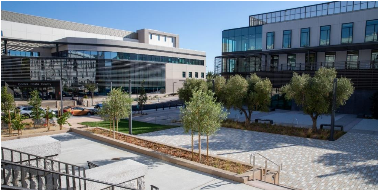
The new Contra Costa County Administration Building, part of the first government project in the world to receive TRUE pre-certification. Photo credit: Contra Costa County staff.
