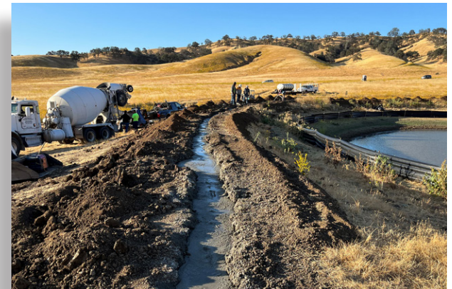
Pond berm repair.
