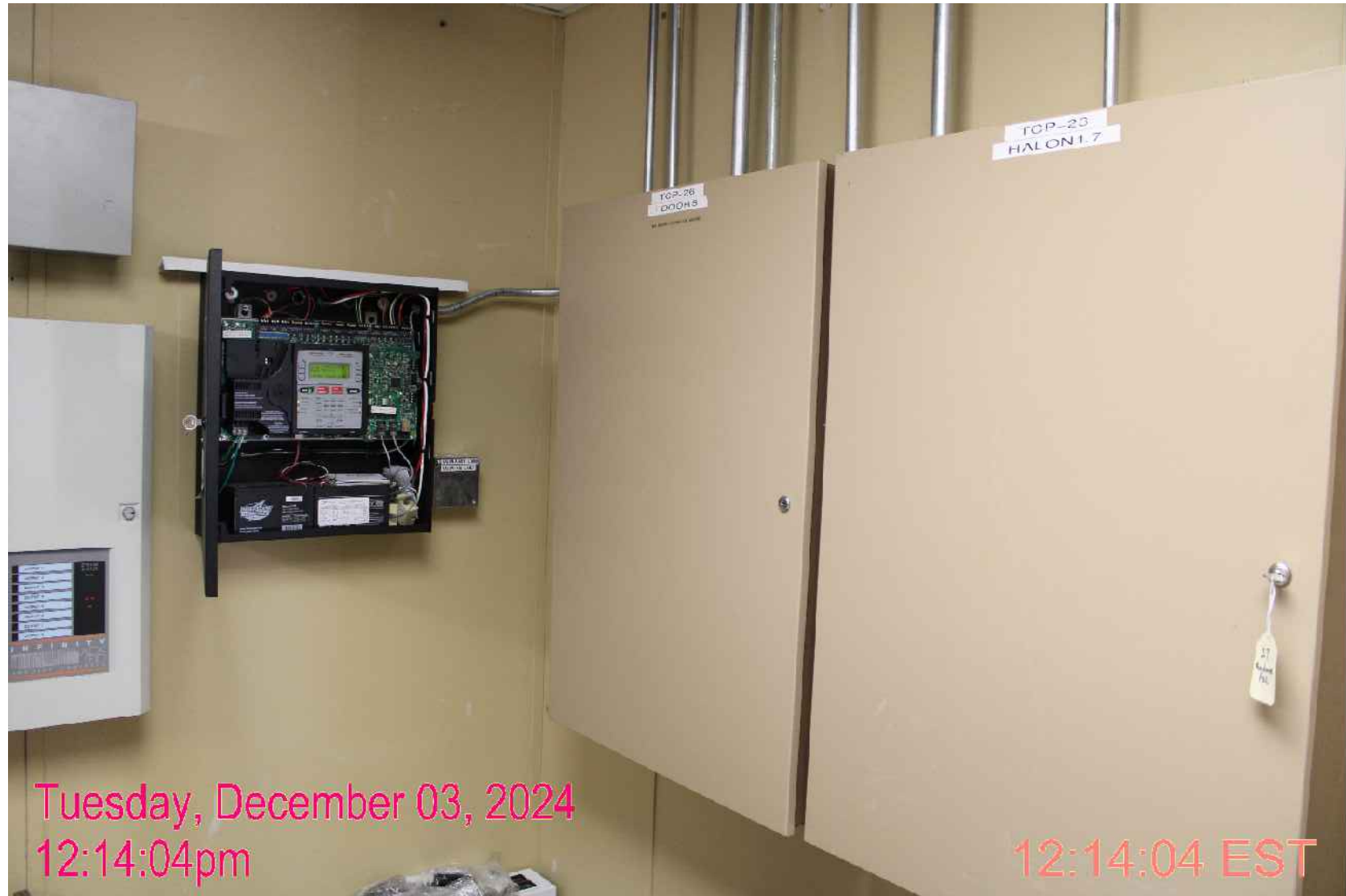
SECURITY AND A/C CONTROL PANELS
