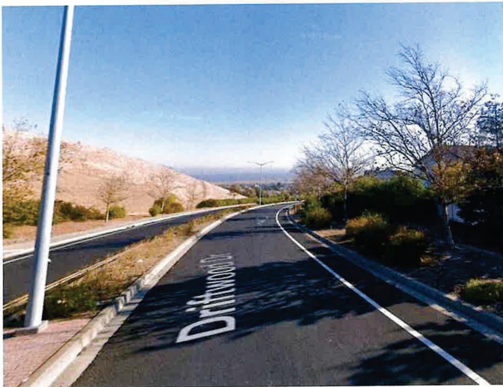
Driftwood Drive between Tradewinds Court/Coastview Court and Steffa Street
