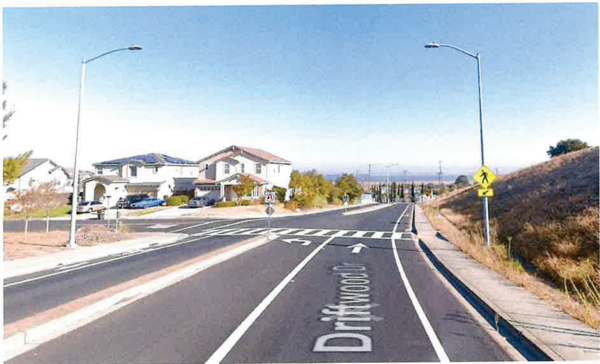
Site 3: Driftwood Drive at Jill Avenue
