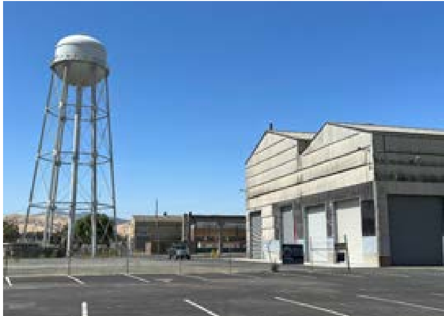
Industrial uses along the Northern Waterfront, like this facility that manufactures commuter trains, provide local jobs and boost the economy.
