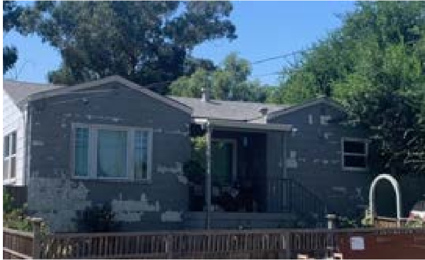
Aging houses may qualify for rehabilitation through the County's Neighborhood Preservation and Weatherization Programs.
