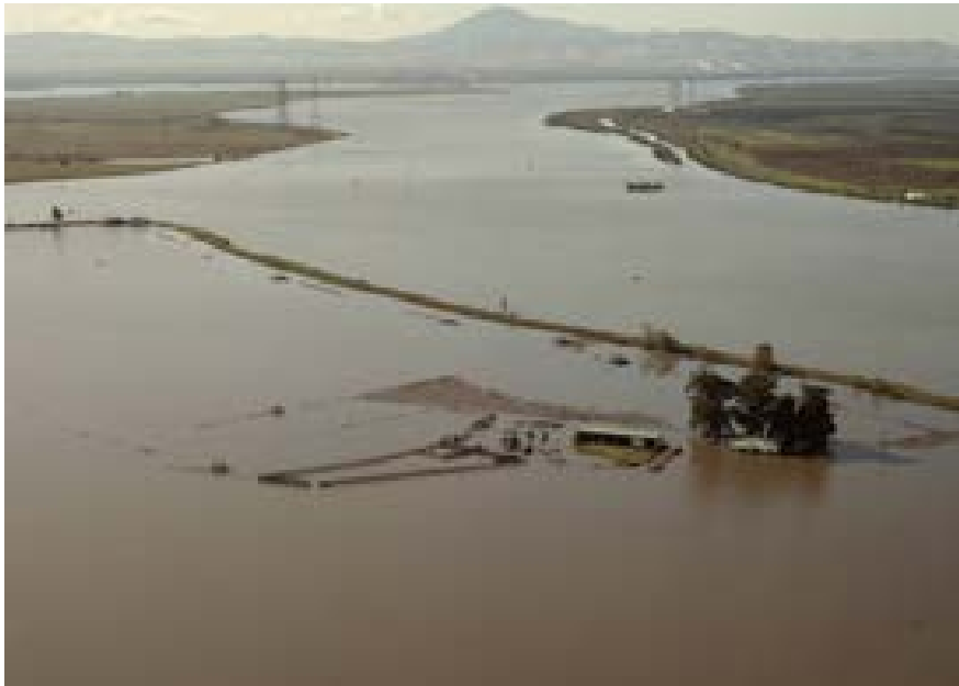
Delta flooding, as occurred on Bradford Island in 1983, is a significant hazard in Contra Costa County. (Credit: California Department of Water Resources)
