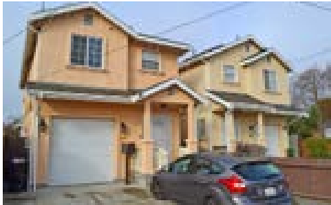
Small lot single-family housing in North Richmond.
