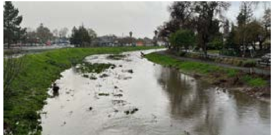
The capacity of Grayson Creek in Pacheco has been increased to protect against flooding
