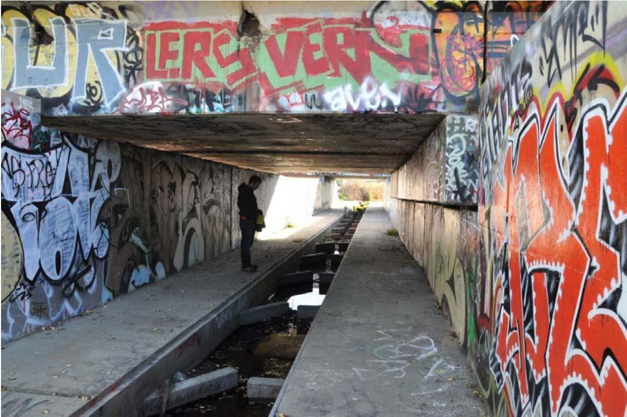
FIGURE 9: CENTER BAY, LOOKING UPSTREAM, AT UPRR CROSSING (NHC 2014).
