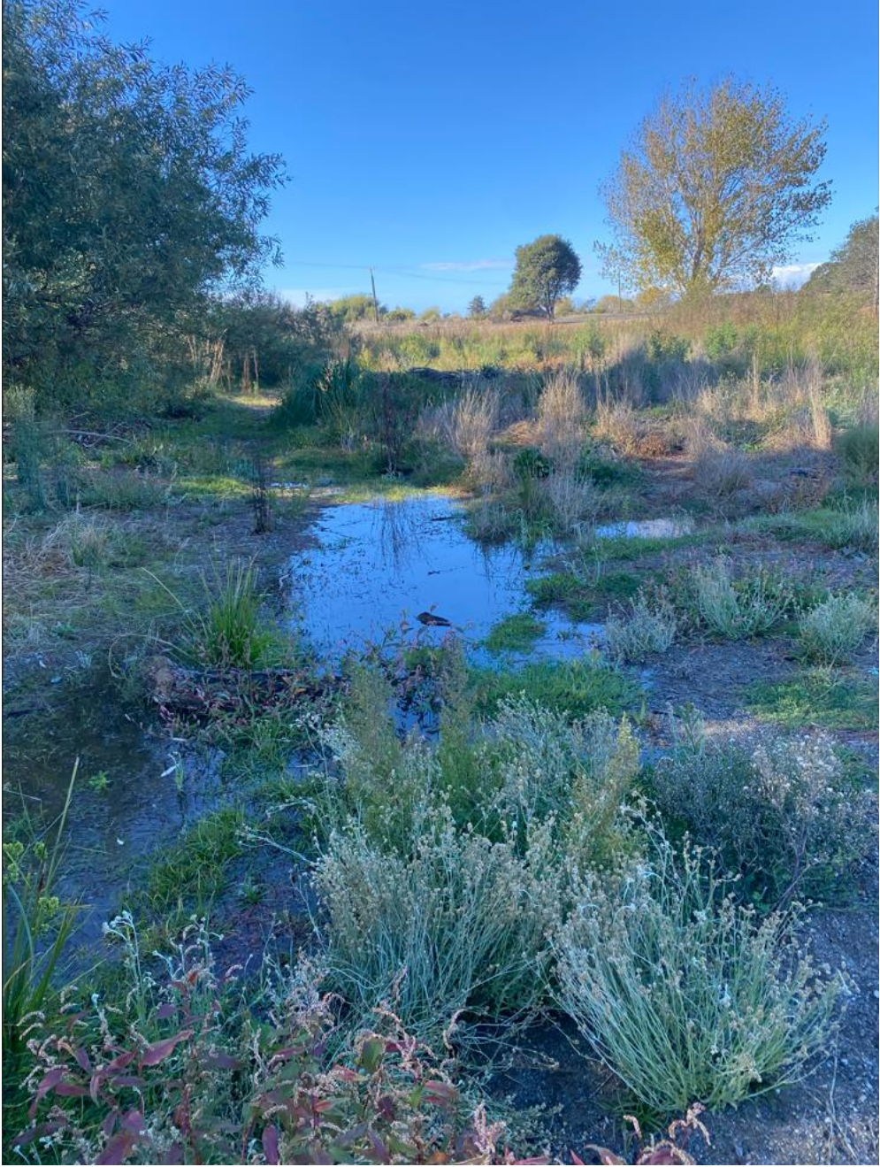
FIGURE 10: SEDIMENT BASIN, LOOKING DOWNSTREAM FROM THE BASE OF FISH PASSAGE STRUCTURE.
