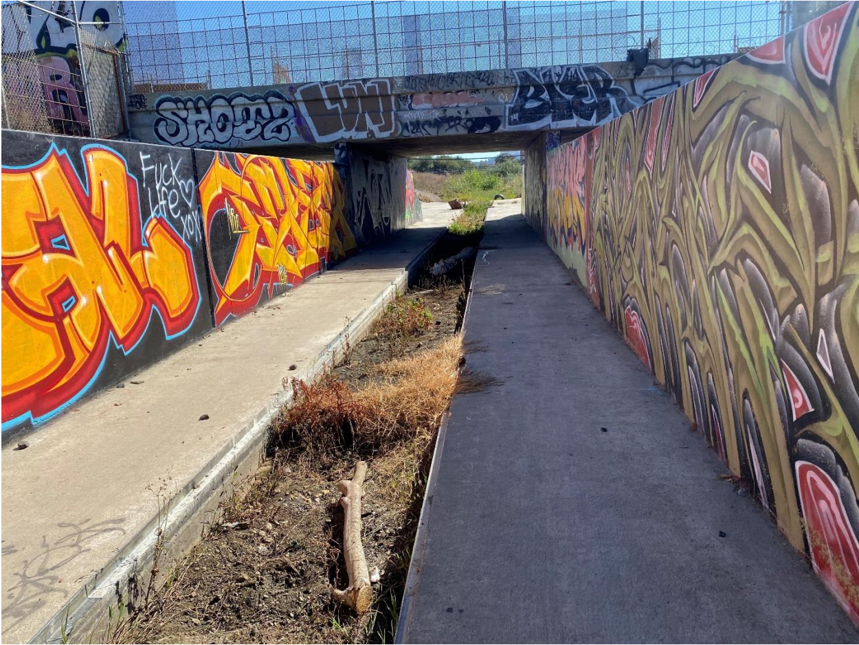
FIGURE 8: FISH PASSAGE STRUCTURE, LOOKING UPSTREAM.
