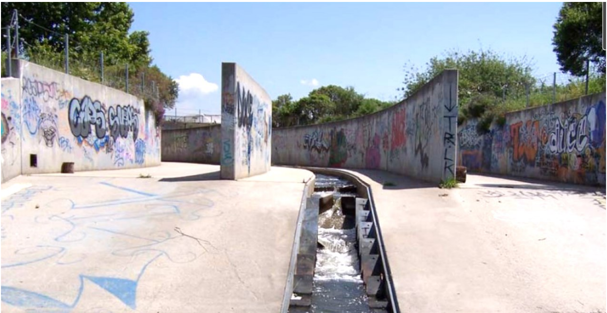
FIGURE 1 - 3: FISH PASSAGE STRUCTURE
