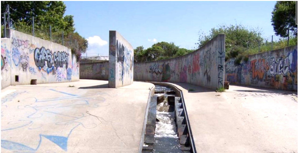
FIGURE 1 - 3: FISH PASSAGE STRUCTURE
