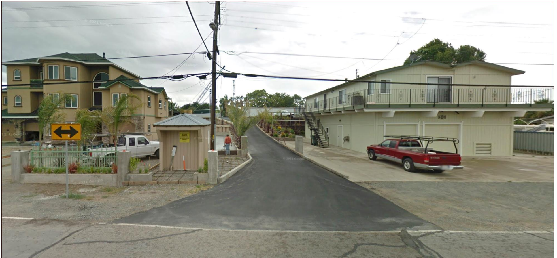
View east from Sandmound Blvd. of 4486 Sandmound Blvd. (right) and 4508 Sandmound Blvd. (left). Small building left of the levee access road is on a separate parcel owned by the Oakley Mutual Water Company. Source: Google Maps, accessed 03/11/2025.
