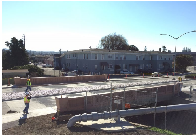
Rodeo Creek Bridge
