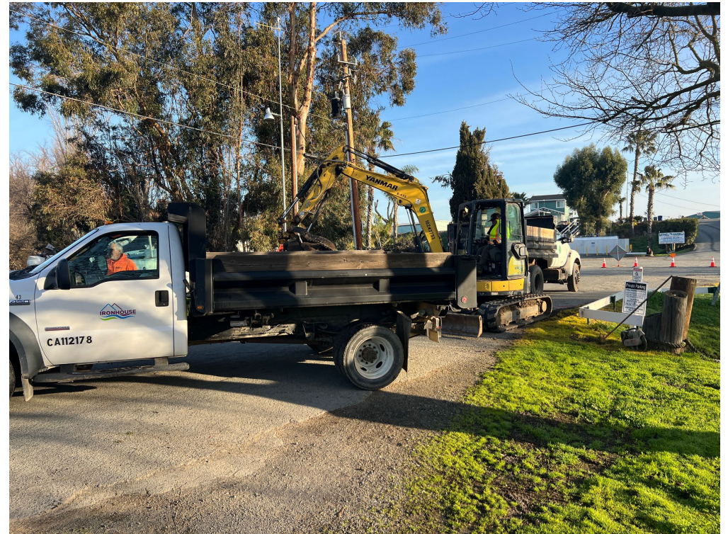
Crew working at Willow 3 LS Site near Harbor Rd.
