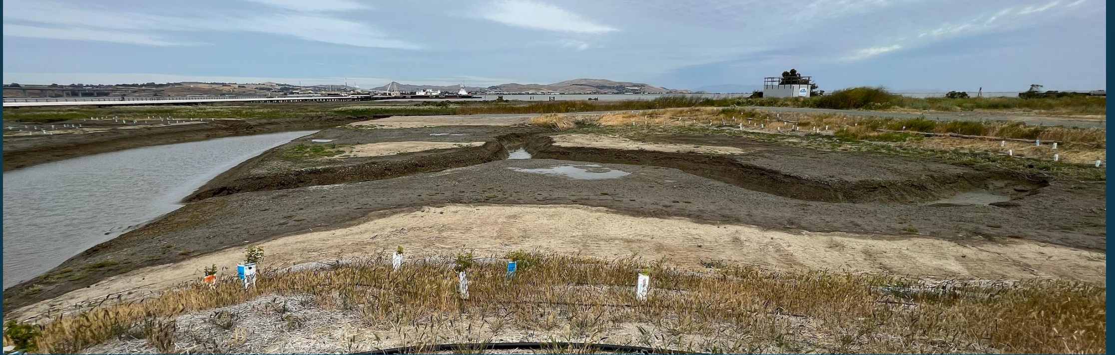
Lower Walnut Creek Restoration Project on May 5, 2022
