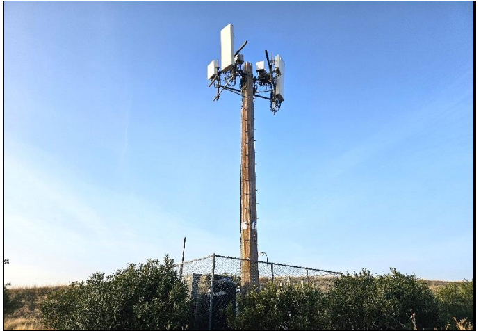
Site Overview from Street View (Diagonal)
