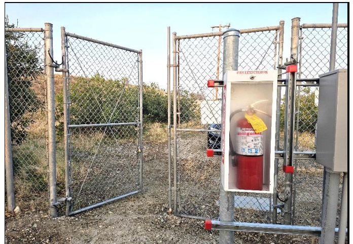
Access Point From Inside
