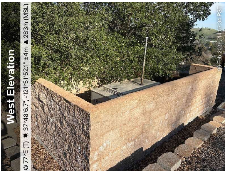
COA 19 Generator enclosure CMU wall in lieu of wood fence for durability
