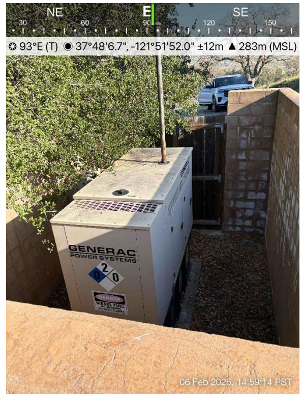
COA 19 Generator enclosure CMU wall in lieu of wood fence for durability
