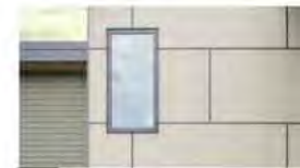
3 FIBER CEMENT BOARD W/ RAIN SCREEN SYSTEM JAMES HARDIE COLOR TO MATCH A OR D
