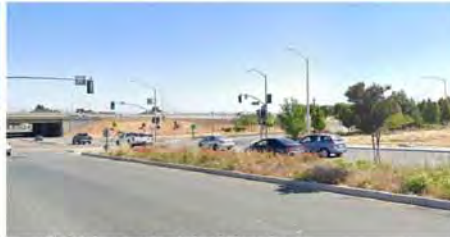
B-VIEW NORTH ON BAILEY RD
