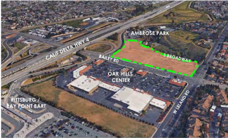
AERIAL VIEW LOOKING NORTHEAST
