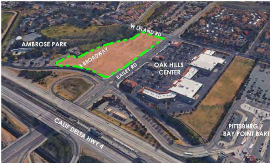
AERIAL VIEW LOOKING SOUTHEAST
