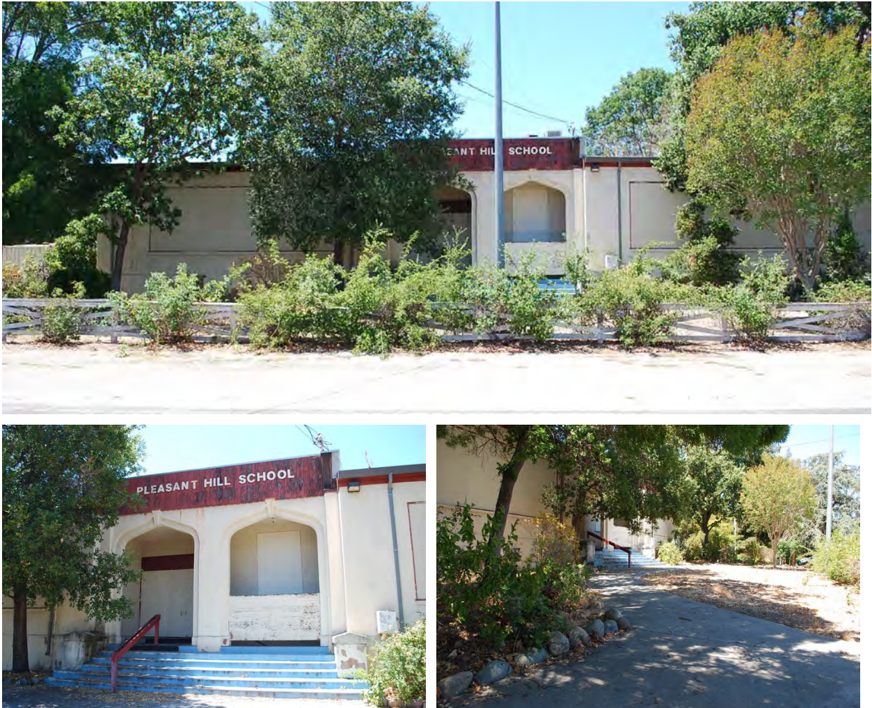
Figure 3: Exterior, Main Façade. Above: Main façade, looking west. Lower left: Entrance steps and arch detail. Lower right: Approach to entrance from half-oval drive, looking north.
