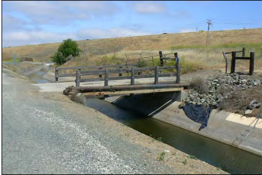
Photograph 4: 20'x25' concrete slab bridge with wooden railing, resting on concrete abutments, crossing Contra Costa Canal, facing northwest, May 30, 2009. (Map Reference # 2)
