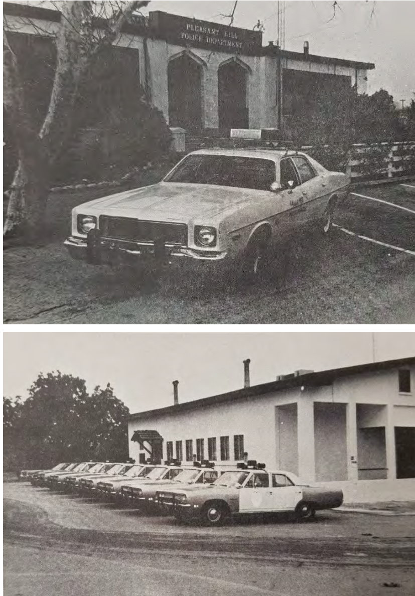
Figure 15: Pleasant Hill Police Department, circa 1970. Above: front façade. Note shortening of eaves and removal of parapet. Below, rear façade. On file, Pleasant Hill Historical Society.
