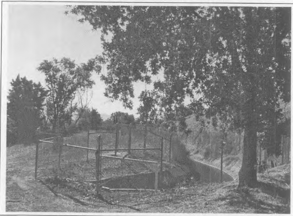
Photograph 5. Area of canal entering siphon to carry water under SR4, 9/20/02, Camera facing south.
