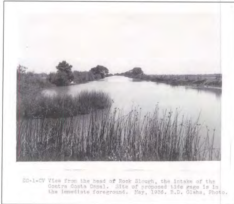
Photograph 52. Photograph caption reads: "CC-1-CV View from the head of Rock Slough, the intake of the Contra Costa Canal. Site proposed tide gage is in the immediate foreground. May, 1936. B. D. Glaha, Photo." Courtesy: Contra Costa Water District
