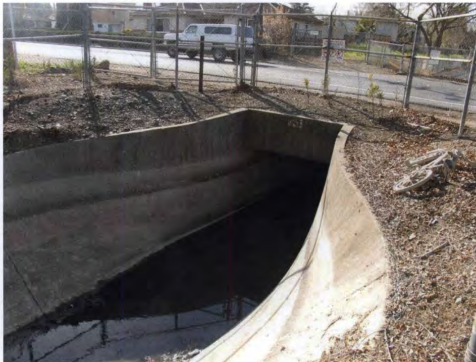
Contra Costa Canal (north of Concord Blvd): looking southeast
