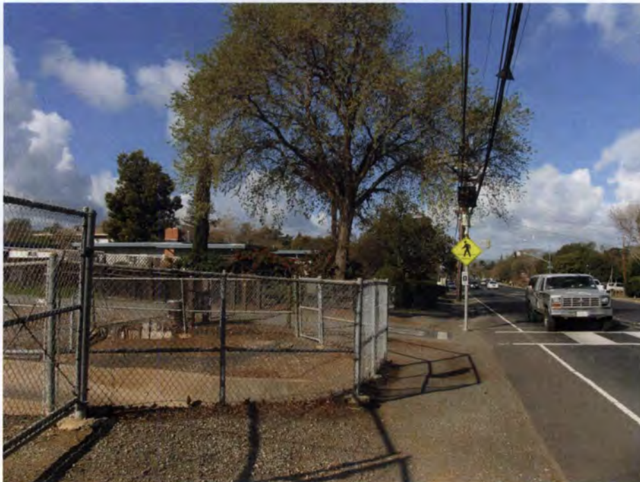
Contra Costa Canal (south of Concord Blvd): looking west
