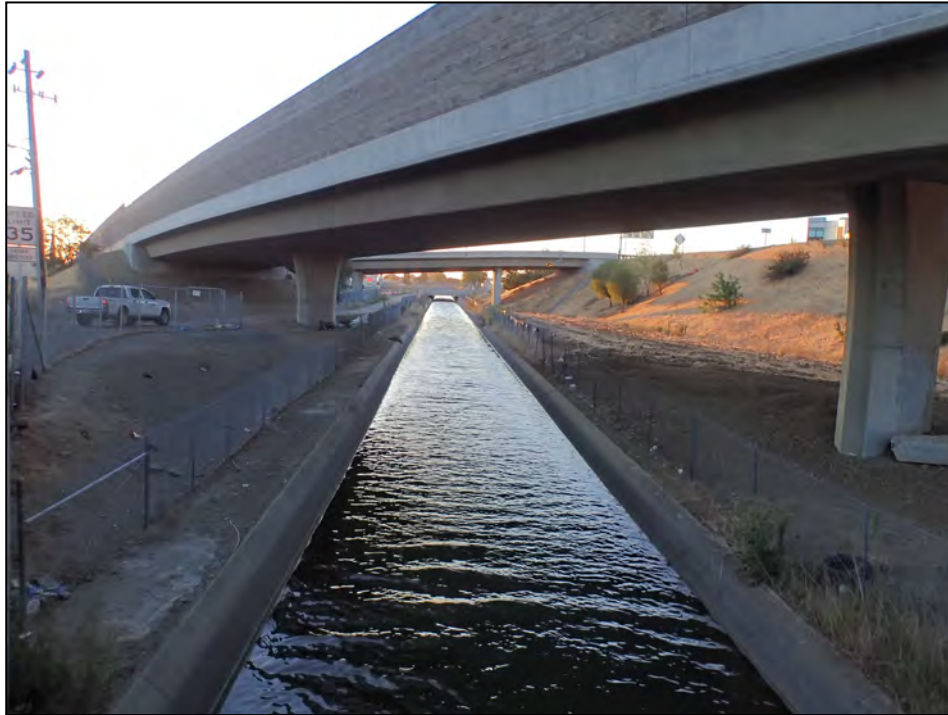
Contra Costa Canal at Alves Lane/Canal Road bridge. View east and upstream of canal LSA photograph, 8.10.2021.
