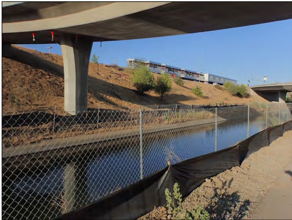
Contra Costa Canal. View northwest across Canal toward SR-4. LSA photograph, 8.11.2021.
