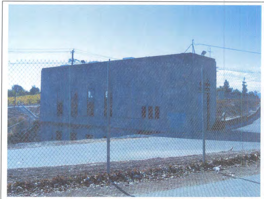
Photograph 57. Pumping Plant No. 2, milepost 4.72, camera facing southwest, November 9, 2005.
