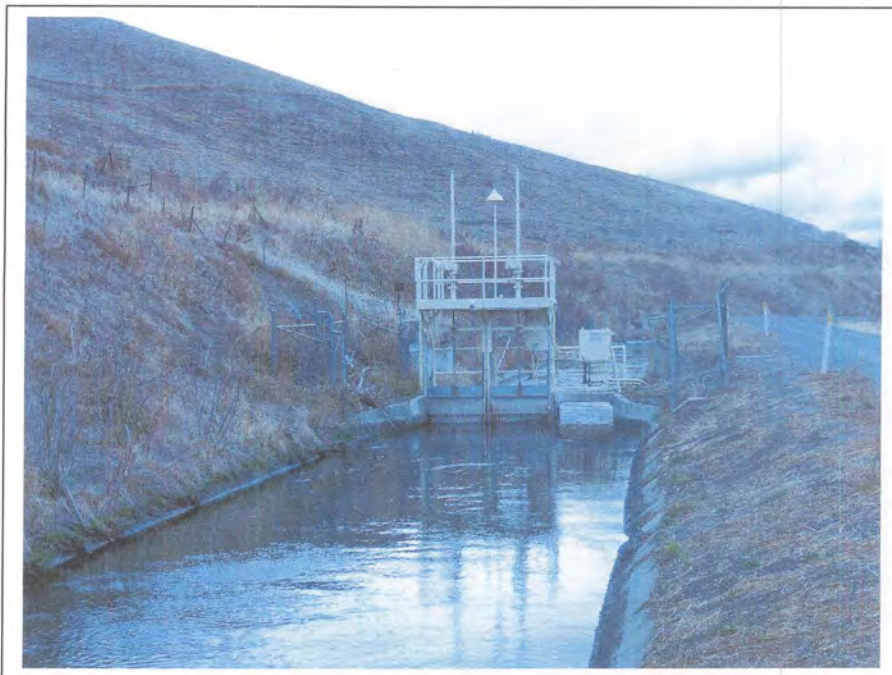
Photograph 69. Check number 7 on the Contra Costa Canal, milepost 23.108, camera facing west, November 7, 2005.
