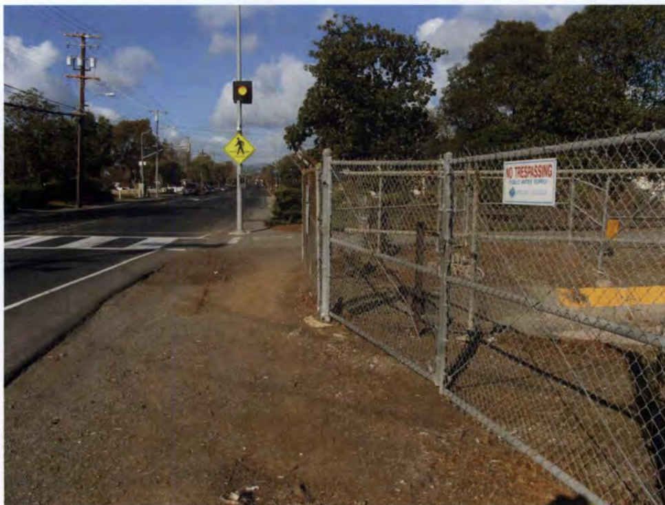
Contra Costa Canal (north of Concord Blvd): looking west
