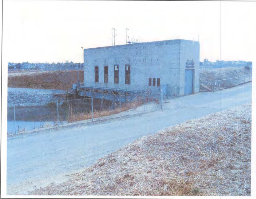
Photograph 56. Pumping Plant No. 1, milepost 3.97, camera facing south, November 1, 2005.
