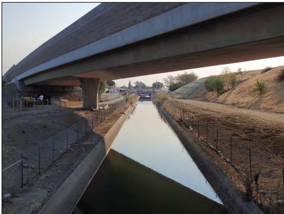
Contra Costa Canal at Alves Lane/Canal Road bridge. View east and upstream of canal LSA photograph, 10.4.2021. Note: off-ramp overpass bridge structure shown in distance in 8.10.2021 is removed.
