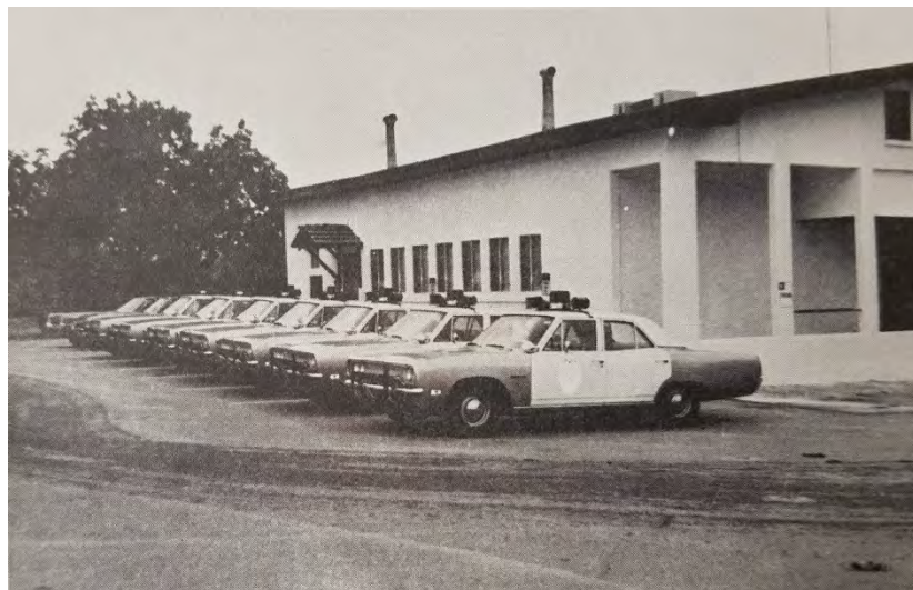
Pleasant Hill Police Department, circa 1970. Above: front façade. Note shortening of eaves and removal of parapet. Below, rear façade. On file, Pleasant Hill Historical Society.
