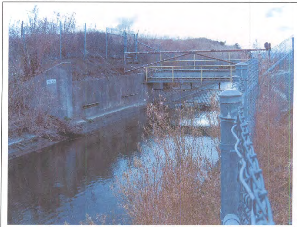
Photograph 60. Bridge abutment, pedestrian bridge and trashrack on the Contra Costa Canal, milepost 24.48, camera facing west, November 7, 2005.
