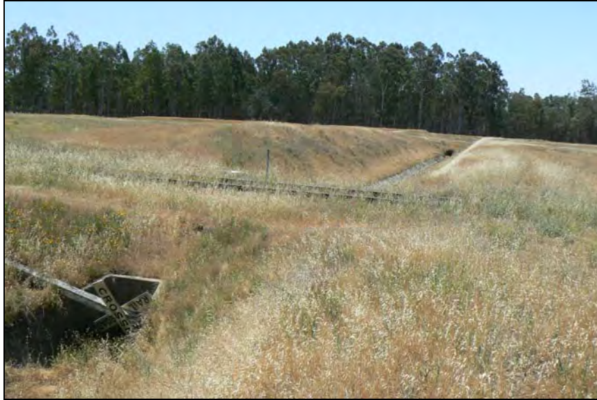
Photograph 14. Railroad tracks run over culvert carrying Clayton Canal, facing west, May 30, 2009. (Map Reference #17)
