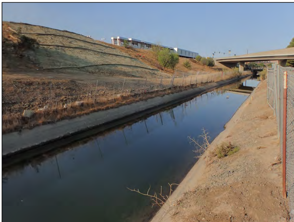
Contra Costa Canal. View northwest across Canal toward SR-4. LSA photograph, 10.4.2021.
