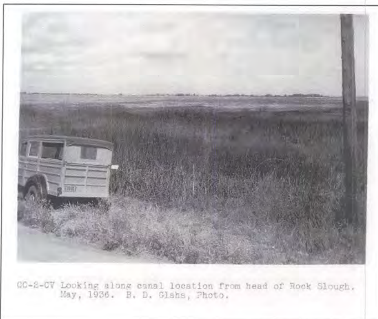
Photograph 53. Photograph caption reads : "CC-2-CV Looking along canal location from head of Rock Slough. May, 1936. B. D. Glaha, Photo." Courtesy: Contra Costa Water District
