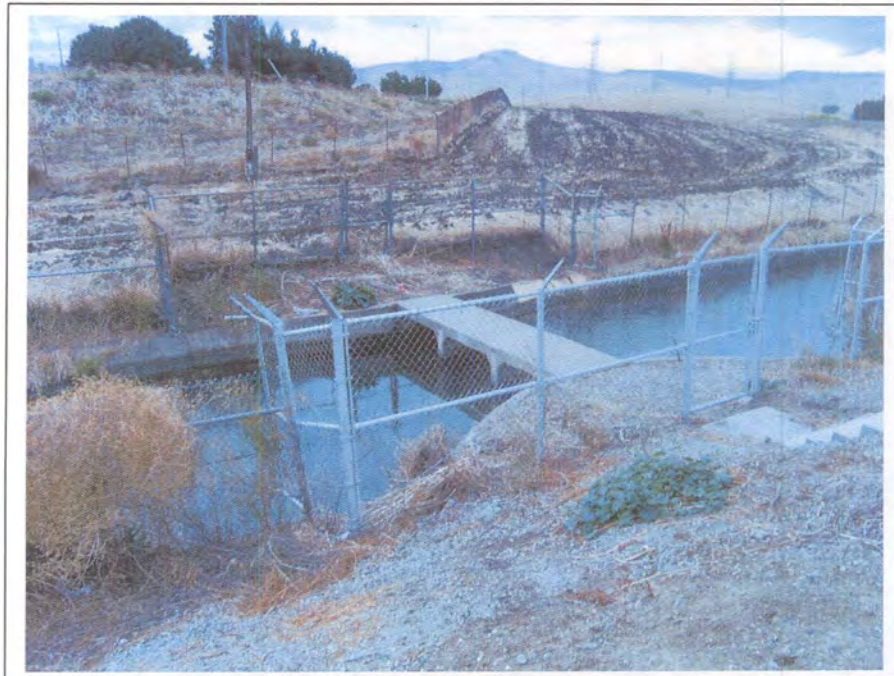
Photograph 73. Typical inactive check structure on the Contra Costa Canal, milepost 17.17, camera facing west, November 7, 2005.
