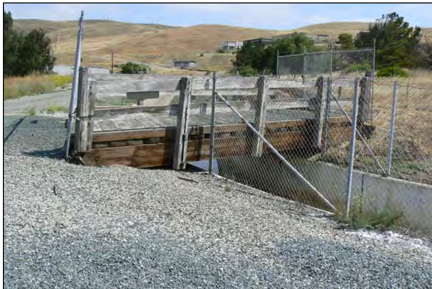
Photograph 3: Farm Bridge, 25' timber beam bridge and railing, crossing Contra Costa Canal, facing north-northeast, May 30, 2009. (Map Reference #1)
