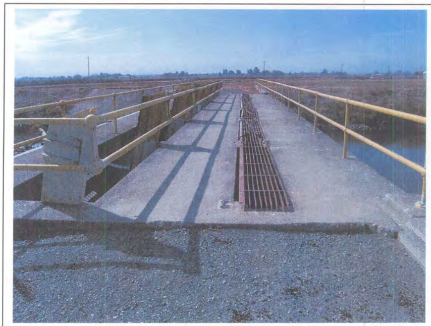
Photograph 55. Deck of the intake trashrack, milepost 0.12, camera facing northwest, November 1, 2005
