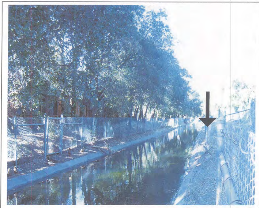
Photograph 76. An example of a typical turnout structure on the Contra Costa Canal, milepost 40.15, camera facing northwest, November 22, 2005.
