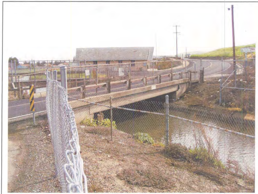
Photograph 63. Typical unaltered bridge over the Contra Costa Canal, showing bridge 28C0376 at Canal Road, milepost 43.07, January 27, 2005.
