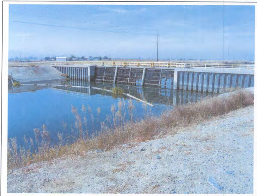
Photograph 40. Intake Trashrack on the Contra Costa Canal, milepost 0.12, camera facing west, November 1, 2005.
