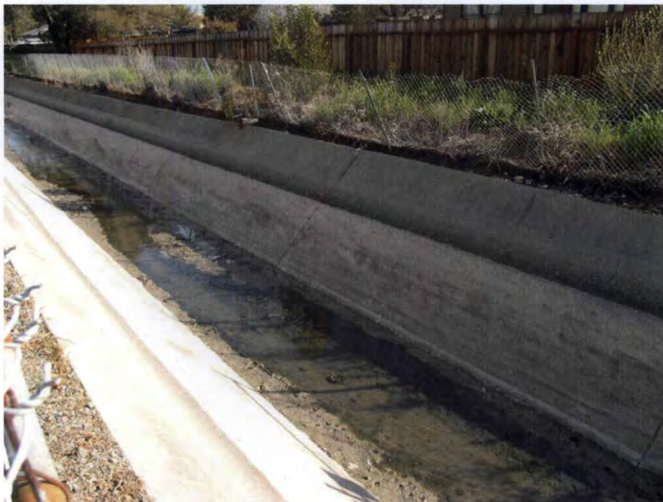
Contra Costa Canal (north of Concord Blvd): looking northeast
