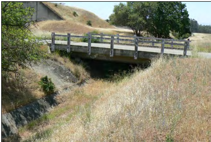
Photograph 11. 20'x30' Steel girder bridge with concrete deck and wooden railings, carrying 11 th Street across the Clayton Canal, facing west, May 30, 2009. (Map Reference #14)
