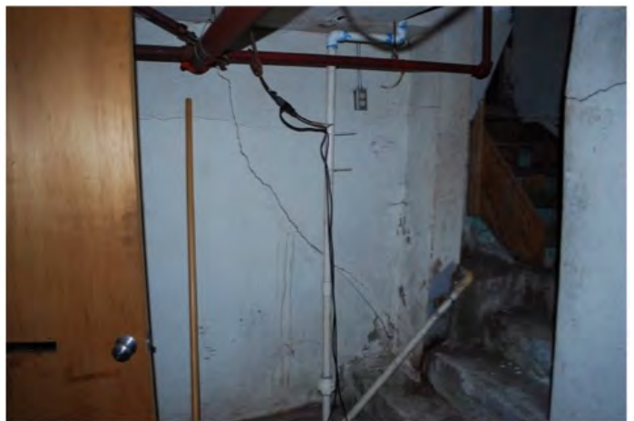
Basement. Left: General view. Right: Stairs up, showing cracked and buckled walls.
