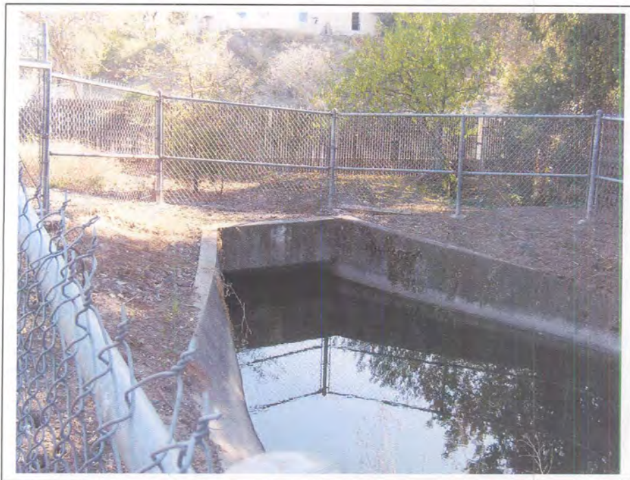
Photograph 78. Example of a typical siphon on the Contra Costa Canal, spanning Walnut Creek, milepost 37.88, camera facing east, November 21, 2005.
