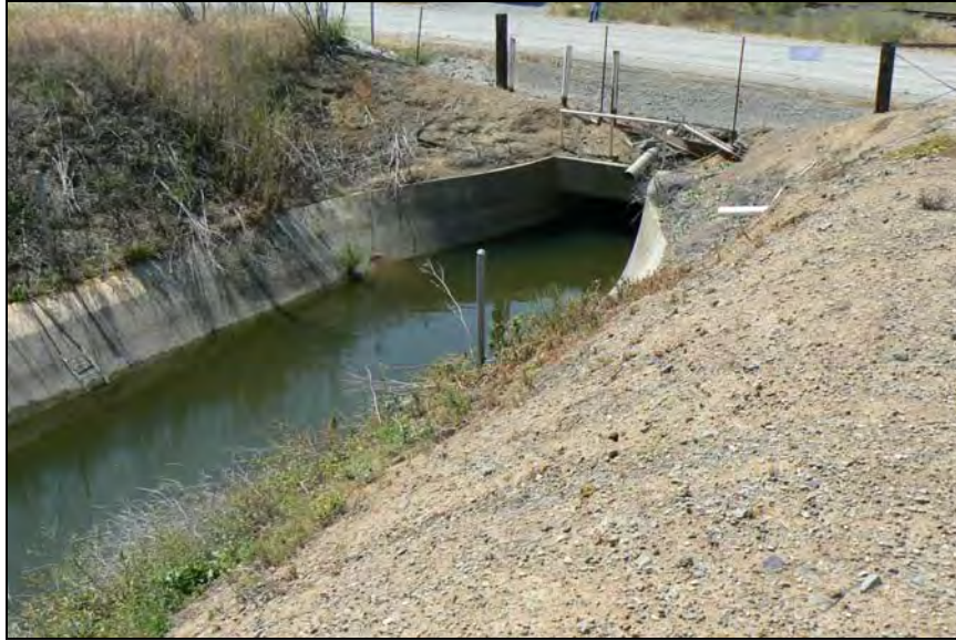
Photograph 2. Contra Costa Canal Culvert below Kinne Road, facing west, May 30, 2009. (Map Reference #4)
