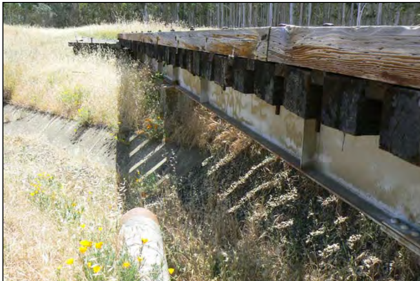
Photograph 15. Railroad bridge, steel girders welded together with timber ties resting on concrete abutments, facing south, May 30, 2009. (Map Reference #18)
