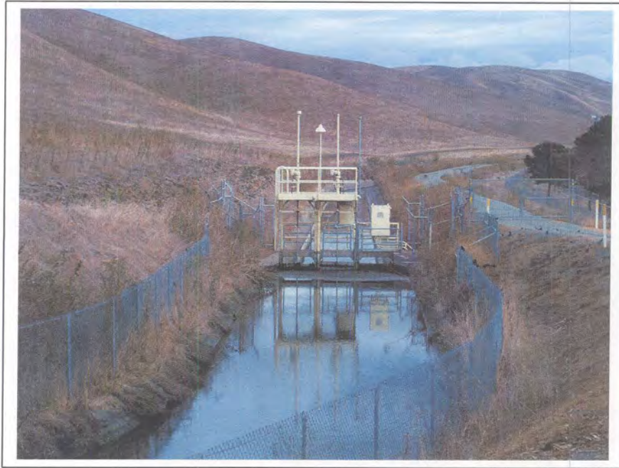
Photograph 70. Check number 8 on the Contra Costa Canal, milepost 26.385, camera facing west, November 7, 2005.
