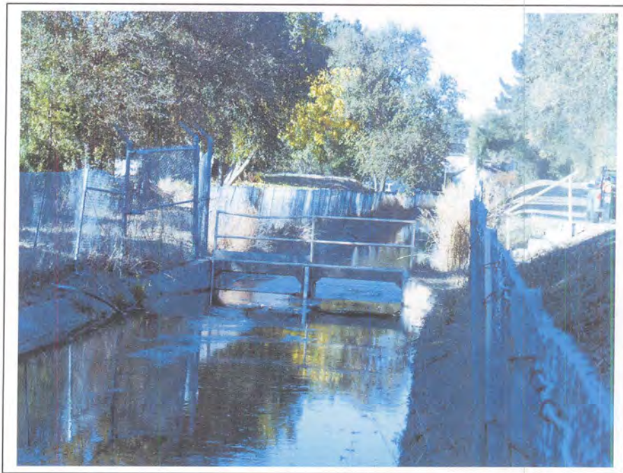
Photograph 74. Typical inactive check on the Contra Costa Canal (Check No. 19 shown), milepost 40.29, camera facing west, November 22, 2005.
