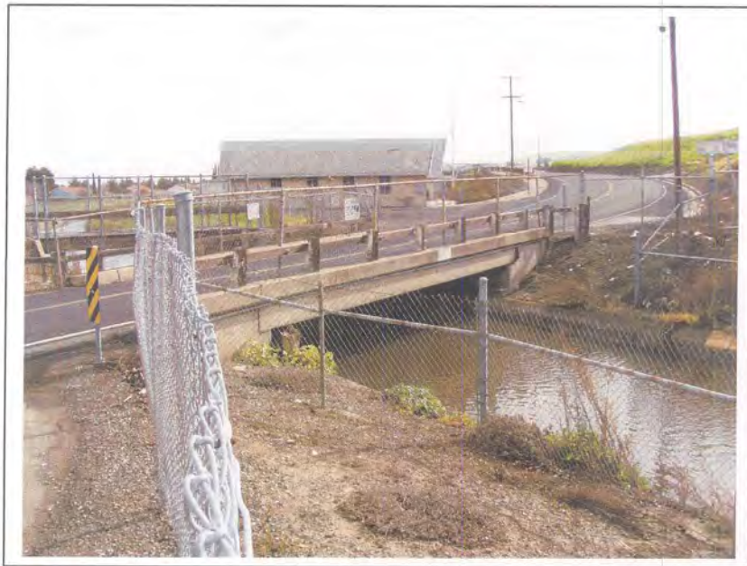
Photograph 42. Typical bridge over the Contra Costa Canal, showing bridge 28C0376 at Canal Road, milepost 43.07, January 27, 2005.
