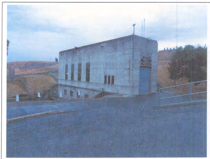
Photograph 59. Pumping Plant No. 4, milepost 7.05, camera facing west, November 7, 2005.
