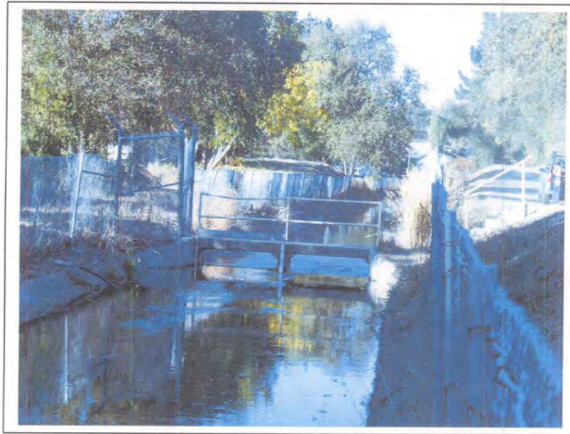
Photograph 44. Typical inactive check on the Contra Costa Canal (Check No. 19 shown), milepost 40.29, camera facing west, November 22, 2005.
