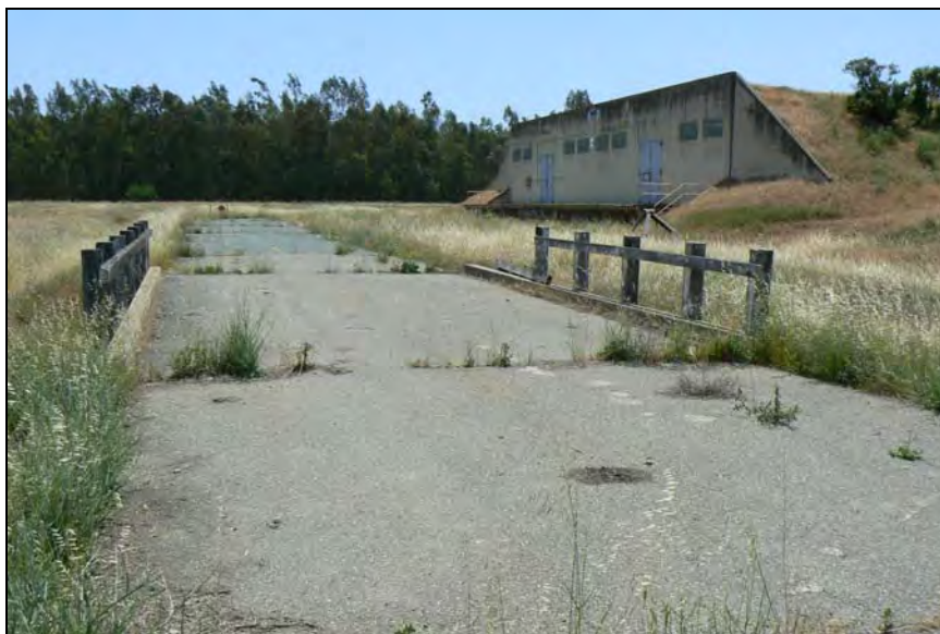
Photograph 13. 20'x30' Steel girder bridge with concrete deck and wooden railings, crossing the Clayton Canal, facing south, May 30, 2009. (Map Reference #16)
