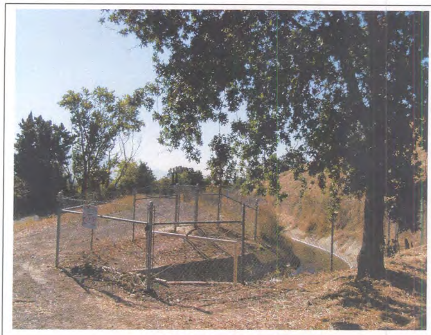
Photograph 83. Area of canal entering siphon to carry water under SR4, September 20, 2002, camera facing south.
