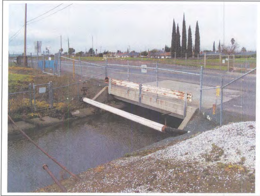
Photograph 64. Typical altered USBR bridge over the Contra Costa Canal, showing bridge 028C0286 at Buchanan Road, milepost 13.84, January 27, 2005.
