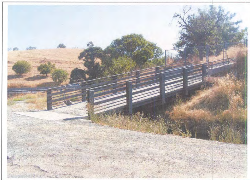
Photograph 61. Modern access bridge, camera facing east, September 12, 2002.
