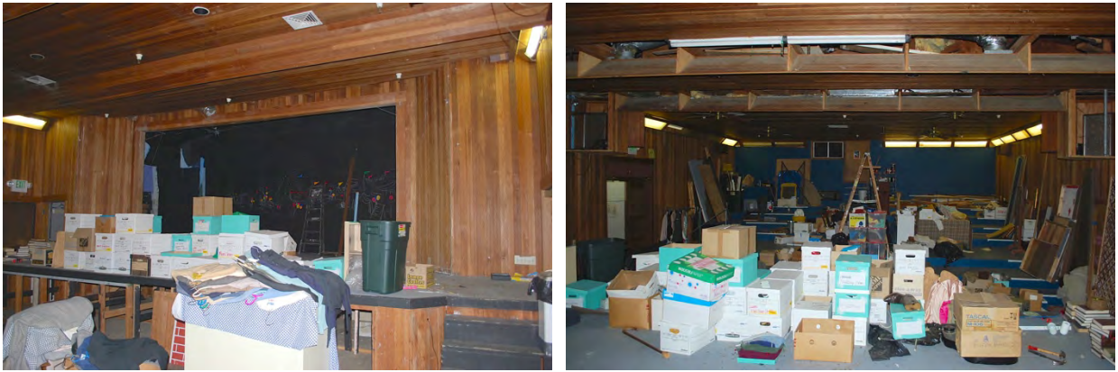
Figure 7: Auditorium. Left: View of stage. Right: Seating area with risers.
