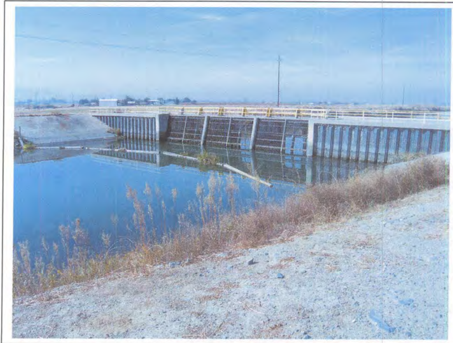
Photograph 54. Intake trashrack, milepost 0.12, camera facing west, November 1, 2005.
