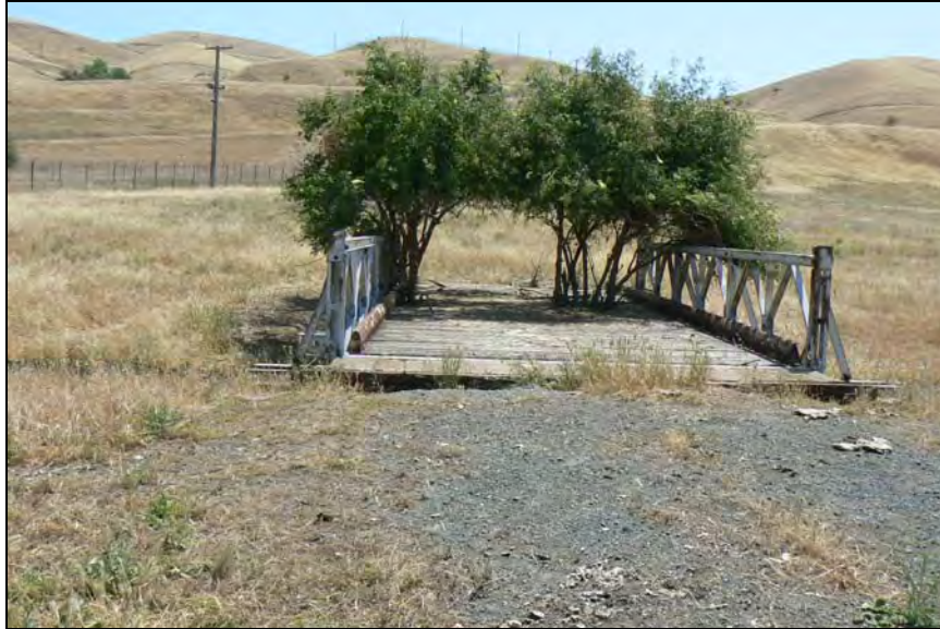
Photograph 10. 20'x30' Farm Bridge, steel "I" beam wooden plank bridge with metal railings, crossing Clayton Canal, facing east, May 30, 2009. (Map Reference #9)
