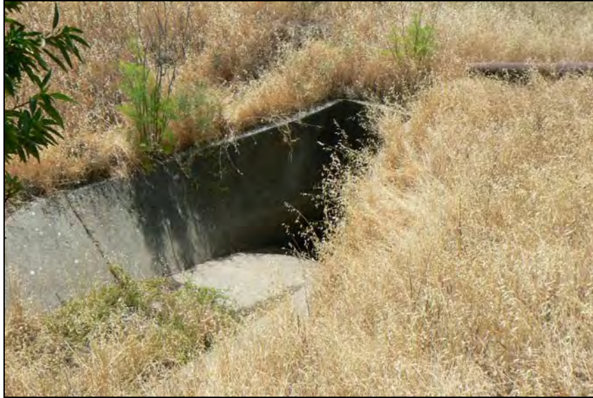
Photograph 18. Concrete culvert carrying Clayton Canal under “S” Street, facing southwest, May 30, 2009. (Map Reference #12)
