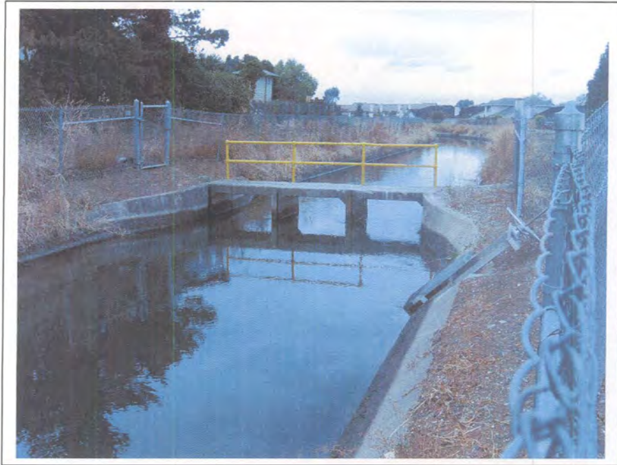
Photograph 72. Typical inactive Check structure on the Contra Costa Canal, milepost 14.86, camera facing west, November 7, 2005.
