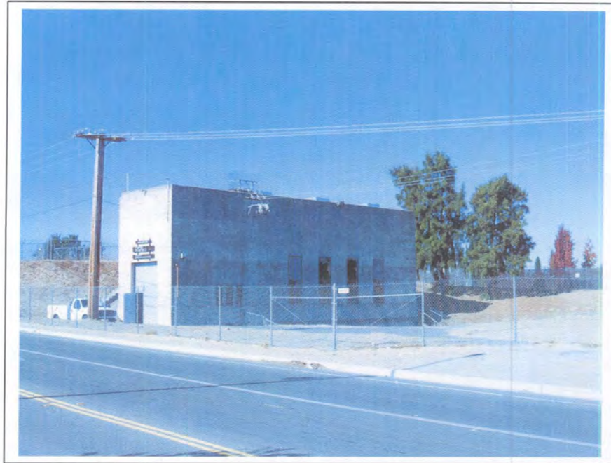
Photograph 58. Pumping Plant No. 3, milepost 5.85, camera facing northwest, November 9, 2005.
