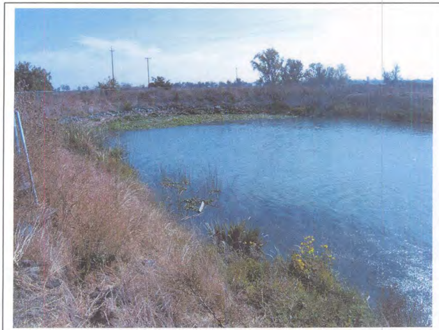
Photograph 77. Example of a typical siphon on the unlined portion of the Contra Costa Canal, milepost 2.05, camera facing southeast, November 1, 2005.
