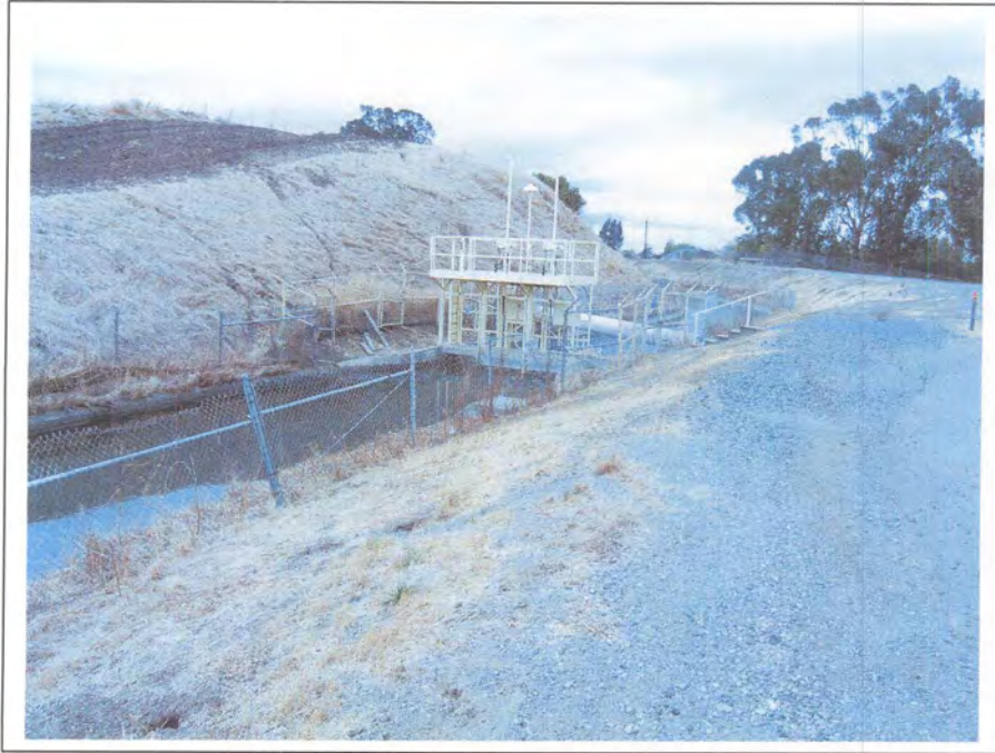
Photograph 68. Check number 6 on the Contra Costa Canal, milepost 20.491, camera facing west, November 7, 2005.
