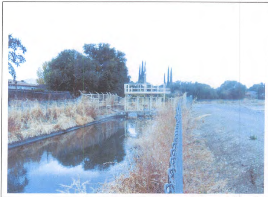
Photograph 66. Check number 4 on the Contra Costa Canal, milepost 15.498, camera facing west, November 7, 2005.
