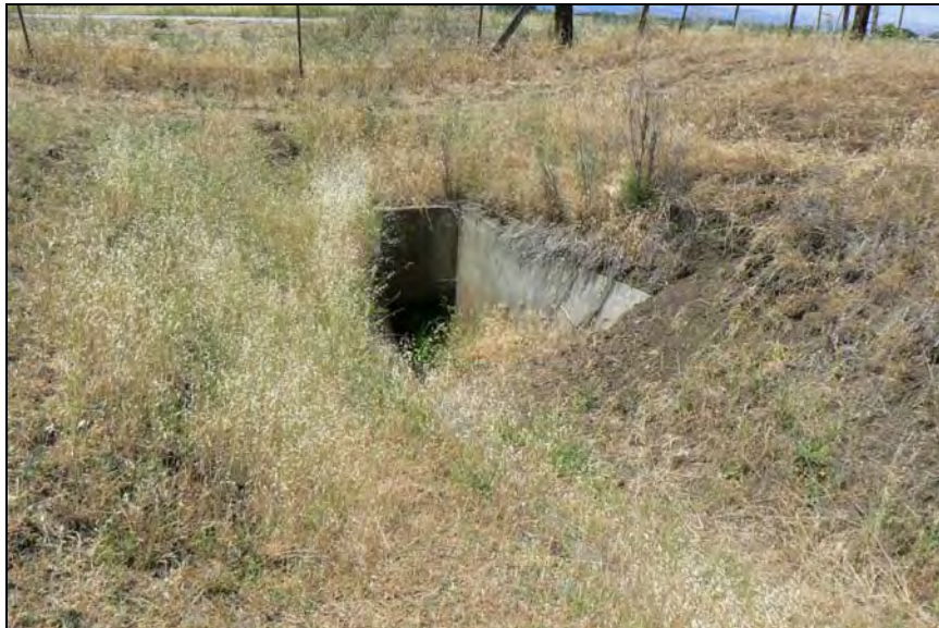
Photograph 17. Concrete culvert carrying Clayton Canal under Kinne Road, facing west, May 30, 2009. (Map Reference #11)
