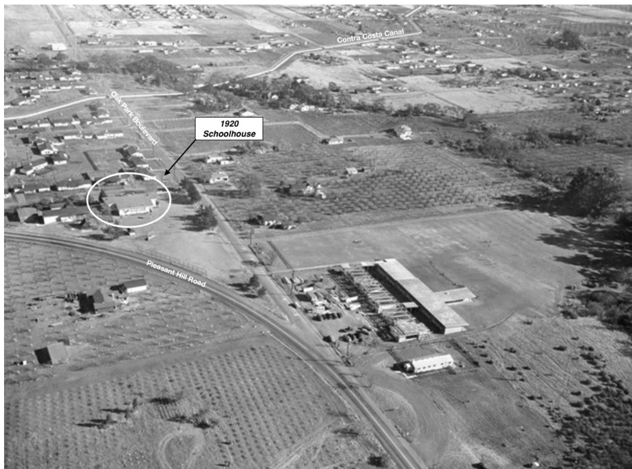
Aerial Photograph of Pleasant Hill School and Vicinity, circa 1950. Looking southeast. Note Contra Costa Canal, new subdivisions, and the new elementary school facility under construction across Oak Park Boulevard. Contra Costa County Historical Society.
