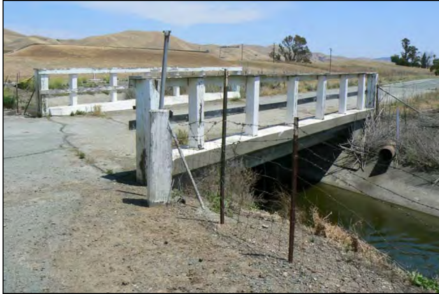
Photograph 6. Concrete tee-beam bridge with wooden railings, crossing Contra Costa Canal, facing southeast, May 30, 2009. (Map Reference #5)
