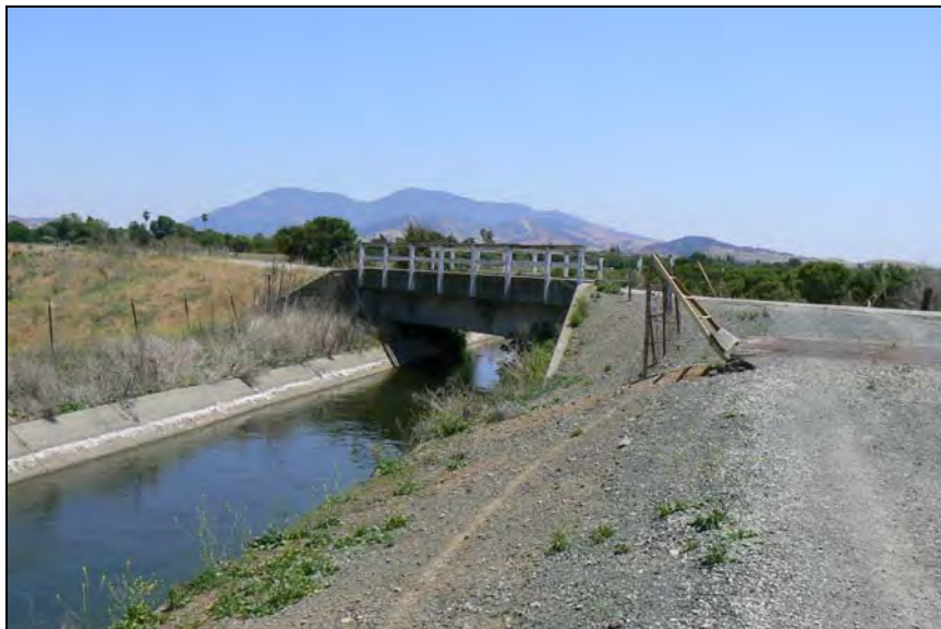
Photograph 9. Concrete tee-beam bridge with wooden railings and concrete abutments, crossing Contra Costa Canal, facing south, May 30, 2009. (Map Reference #8)
