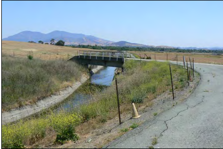
Photograph 8. Concrete tee-beam bridge with wooden railings and concrete abutments, crossing Contra Costa Canal, facing south, May 30, 2009. (Map Reference #7)
