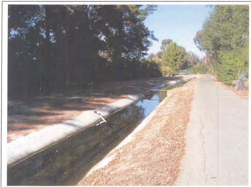
Photograph 91. Typical section of the Ygnacio Canal, approximately milepost 1.44, camera facing east, November 21, 2005.
