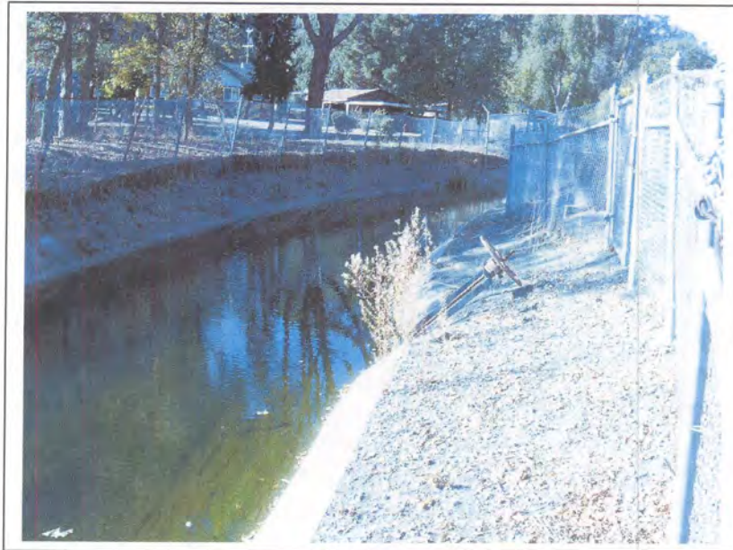
Photograph 45. Typical turnout on the Contra Costa Canal, milepost 39.76, camera facing northwest, November 22, 2005.
