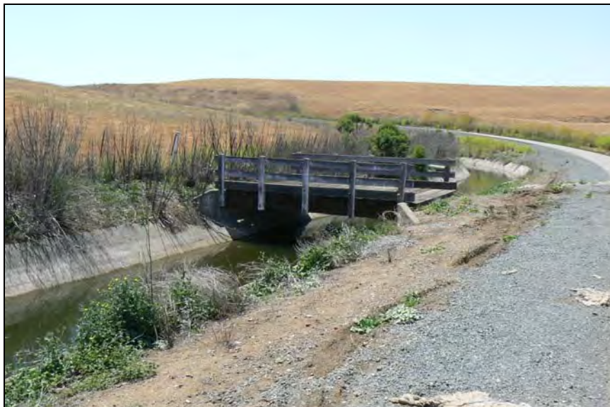
Photograph 7. Farm bridge, timber beam plank bridge with wooden railings, Crossing Contra Costa Canal, facing west, May 30, 2009. (Map Reference #6)
