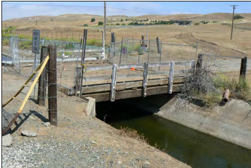
Photograph 5. 16'x30' farm bridge, timber beam plank bridge and wooden railing, crossing Contra Costa Canal, facing north, May 30, 2009. (Map Reference #3)
