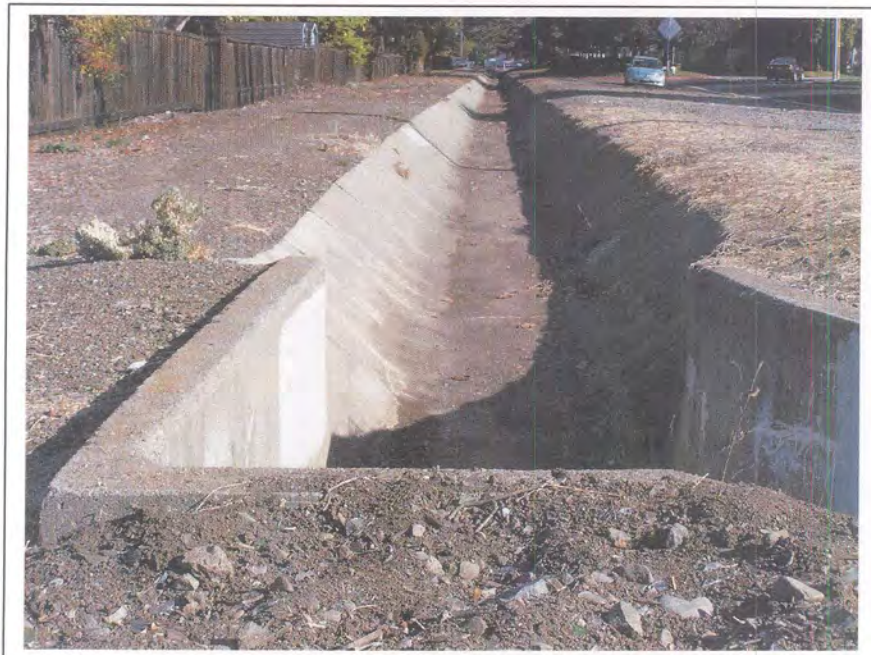
Photograph 87. Detail of segment of the Clayton Canal, at the corner of Denkinger Road and Denkinger Court, camera facing northeast, November 22, 2005.
