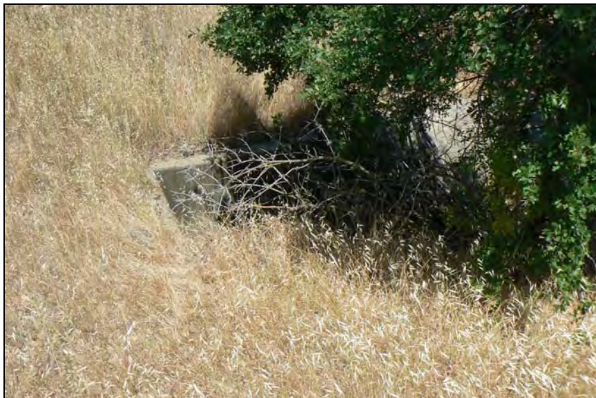
Photograph 19. Concrete culvert carries canal under railroad spur into siphon across Mt. Diablo/Seal Creek, facing west, May 30, 2009. (Map Reference #13)
