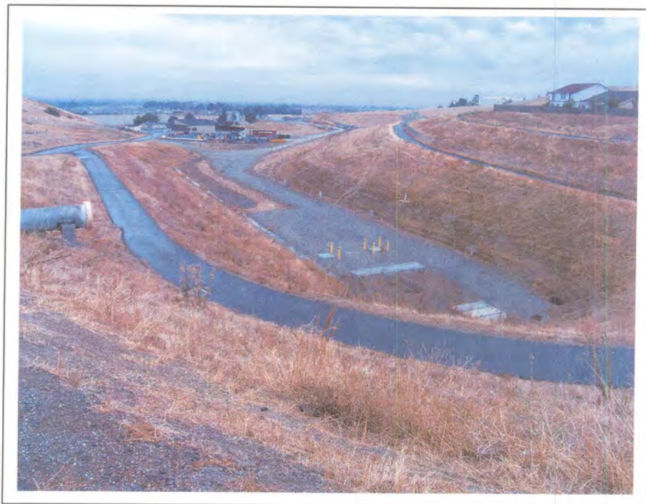
Photograph 80. Tunnel No. 1 on the Contra Costa Canal east of Pumping Plant No. 4, approx. milepost 7.9, camera facing west, November 7, 2005.
