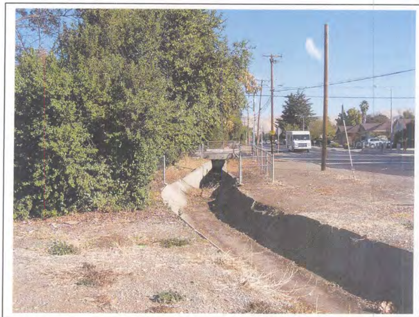
Photograph 50. Typical segment of the abandoned Clayton Canal, one of two branch canals of the Contra Costa Canal, approximately Clayton Canal milepost 4.1, camera facing northeast, November 22, 2005.
