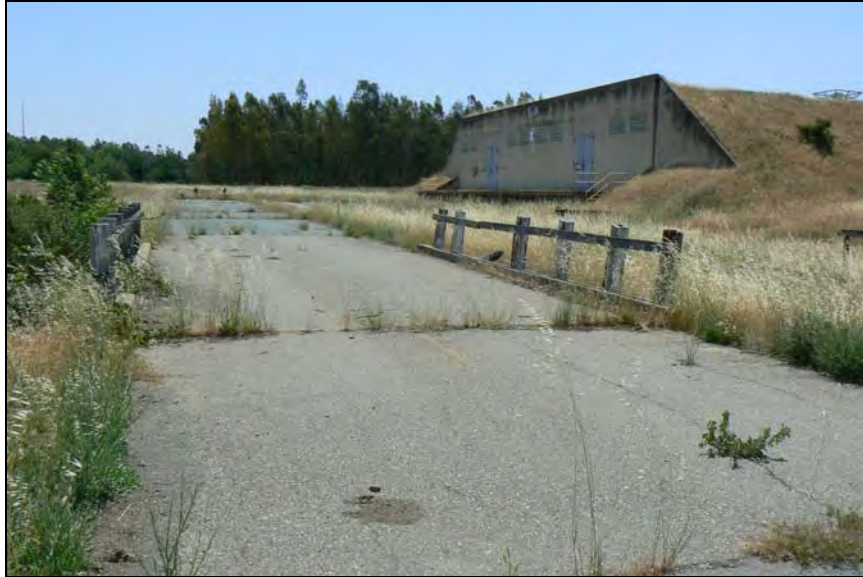
Photograph 12. 20'x30' Steel girder bridge with concrete deck and wooden railings, crossing the Clayton Canal, facing south, May 30, 2009. (Map Reference #15)
