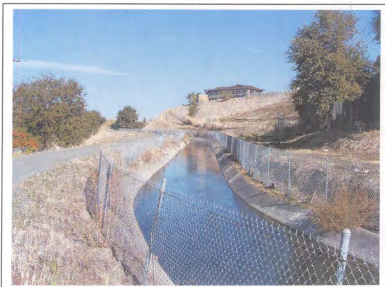
Photograph 47. Typical concrete lined segment of the Contra Costa Canal, milepost 33.25, camera facing northwest, November 22, 2005.
