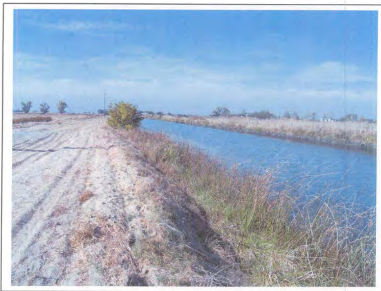
Photograph 46. Typical unlined segment of the Contra Costa Canal, milepost 1.1, camera facing west, November 1, 2005.
