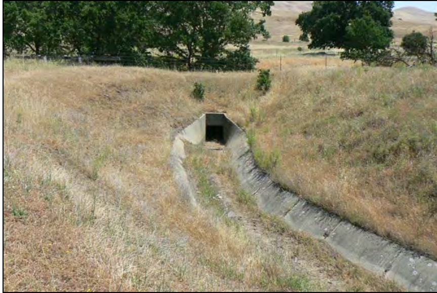
Photograph 20. Concrete culvert carrying Clayton Canal from Mt. Diablo/Seal Creek, facing east, May 30, 2009. (Map Reference #13)
