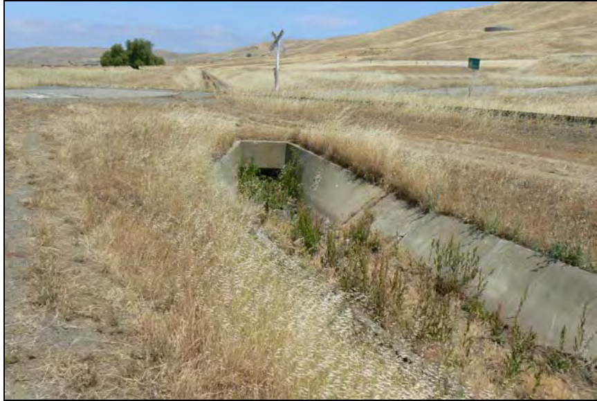
Photograph 16. Concrete culvert carries the Clayton Canal beneath Wildan Road. On the opposite side a railroad spur meets Wildan Road, facing north, May 30, 2009. (Map Reference #10)
