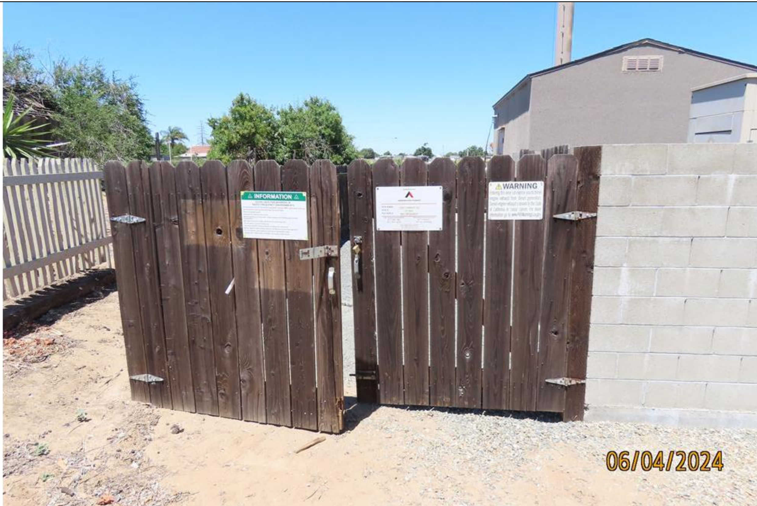
① EXISTING COMPOUND GATE
