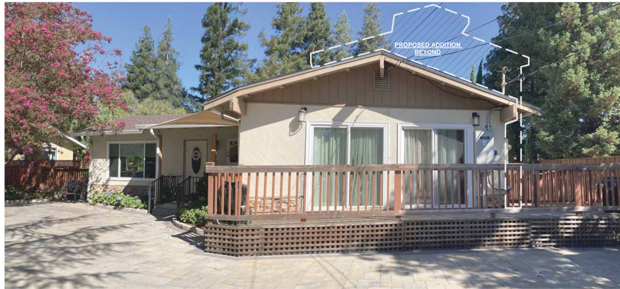
1 PHOTO 1 - FRONT VIEW ALONG WARREN RD SCALE: NTS
