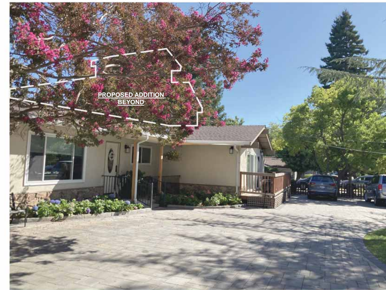
2 PHOTO 2 - FRONT VIEW FACING EAST SCALE: NTS
